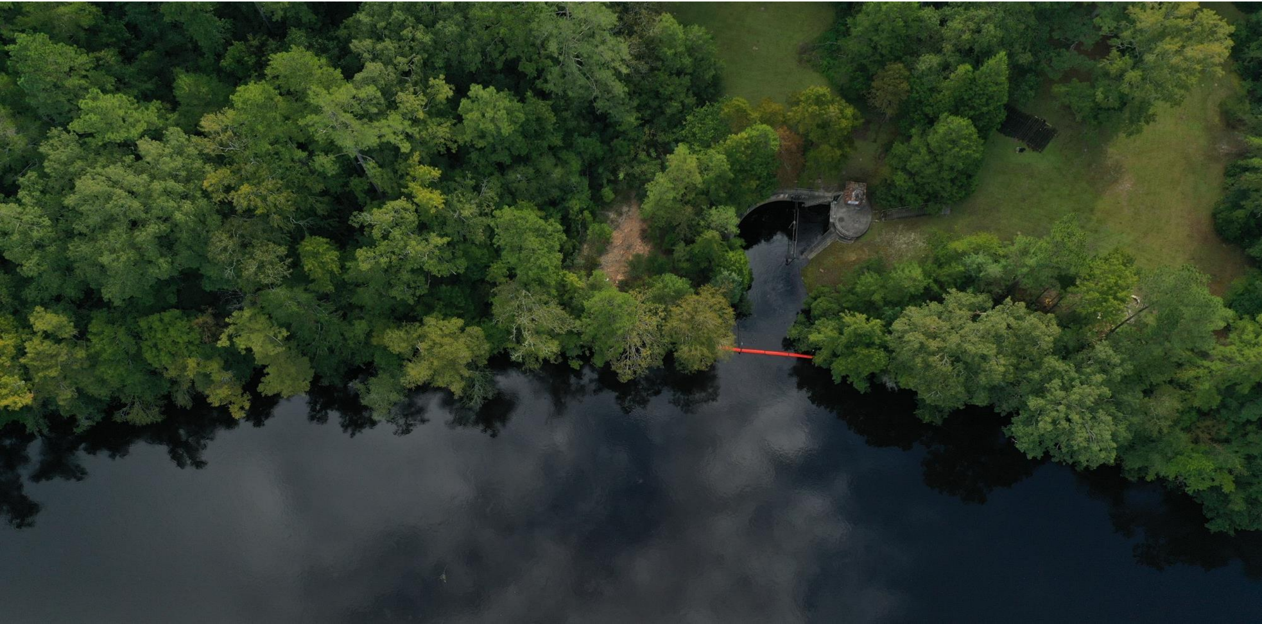
Charleston Water System Intake at Givhans Ferry State Park
