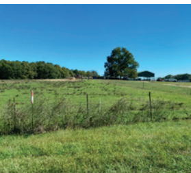
Municipal Reservoir #1 Dam
