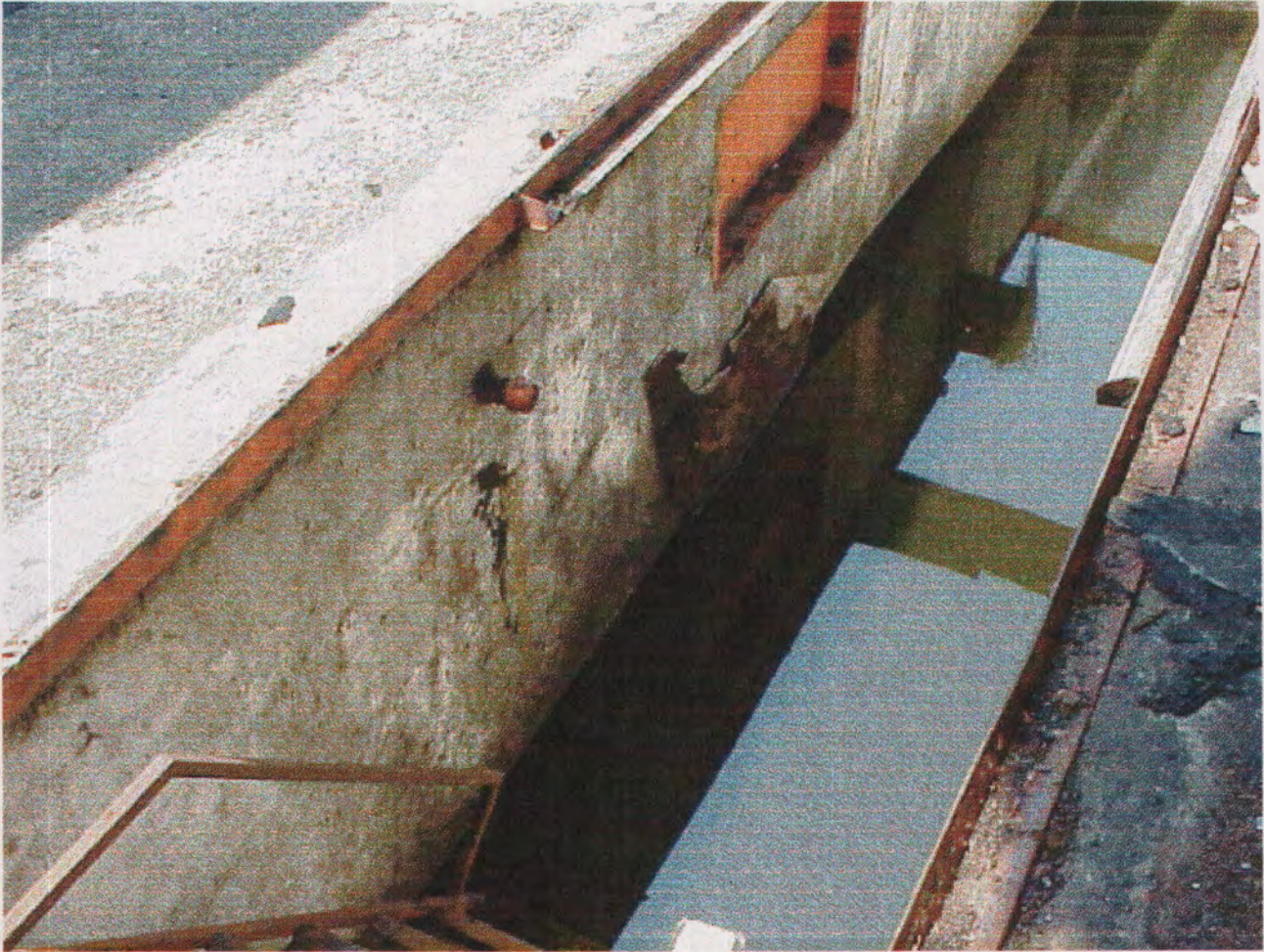
Bay AREA in Back of facility
