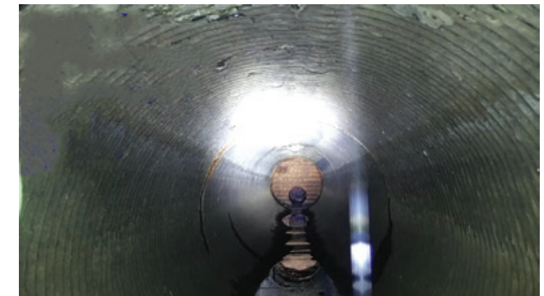
Dam Safety Staff Photo – Camera Inspection of a Spillway Conduit
