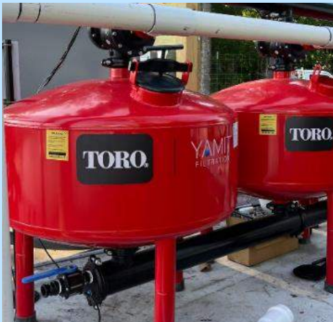
Filter Stations for Water Reuse
