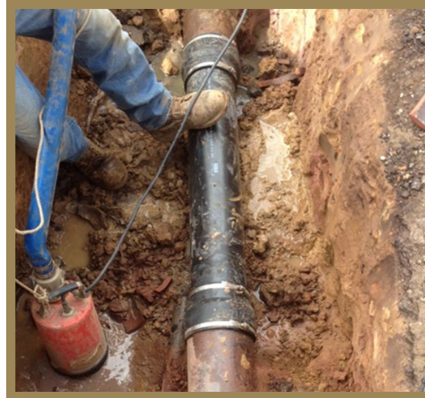
Figure 5.5 Repaired section of sanitary sewer line (Paradise Plumbing)
