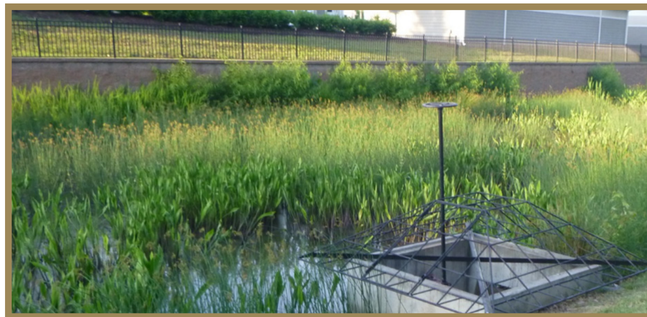
Figure 5.14 Stormwater wetlands clean water well and look attractive (McAdams)
