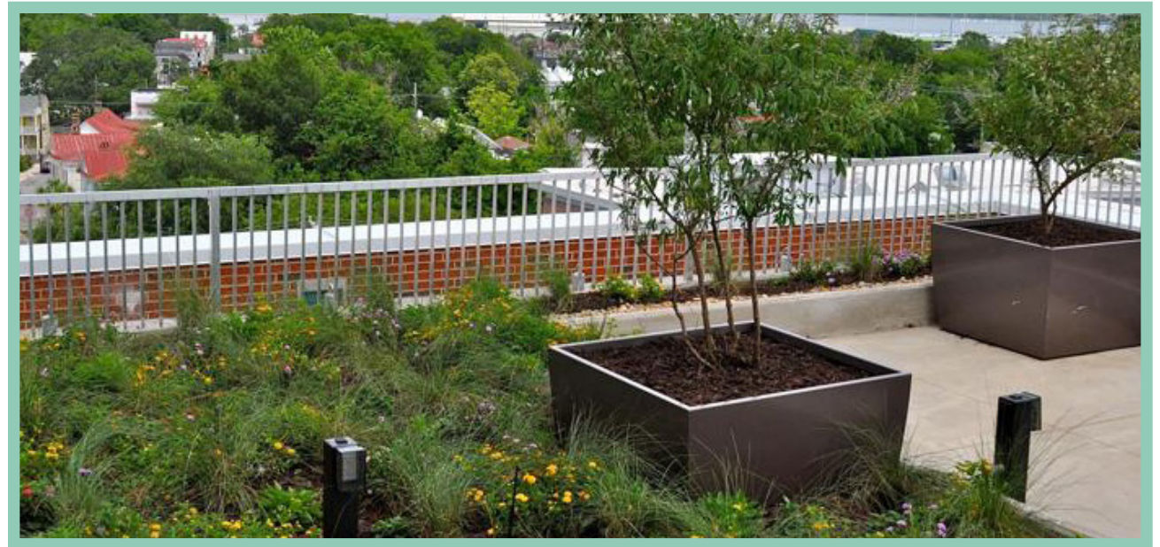
Figure 6.8 A green roof on the rooftop terrace at the SkyGarden Apartment in Charleston, SC (The Post and Courier)
