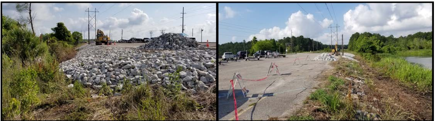
Figure 23. New Riprap to Bushy Park Reservoir Dam and Boat Landing
