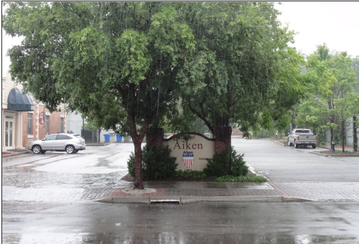
Fig. 28. This image from Aiken, SC demonstrates the ability of a porous asphalt road (right) to quickly infiltrate rain water, in comparison to standard asphalt (left) showing puddles (Source: Calvin Sawyer, Ph.D., Clemson University).
