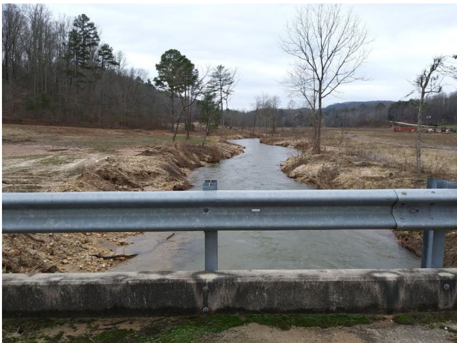
Photo 14. Unstable streambanks and lack of riparian buffer on the North Saluda River
