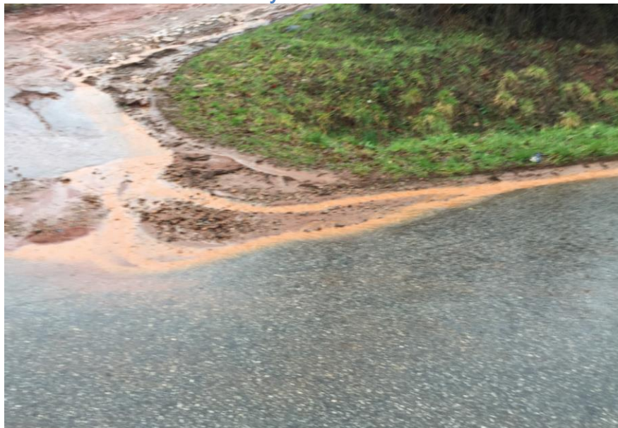
Photo 13. Erosion from a driveway in North Saluda River – Saluda Lake Watershed
