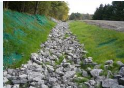
Ditch Stabilization
