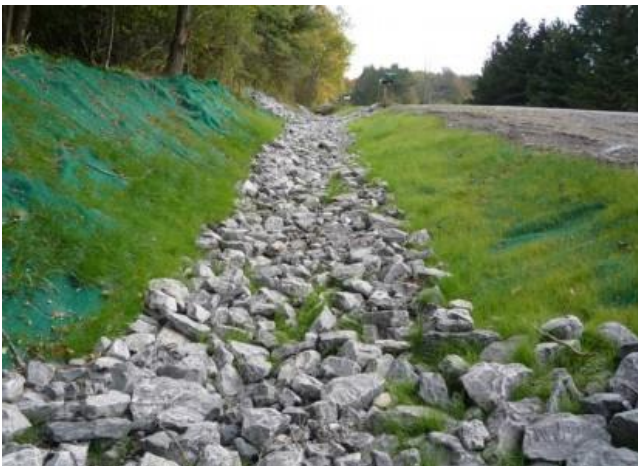
Photo 24. Crop Farm Best Management Practice – Ditch Stabilization
