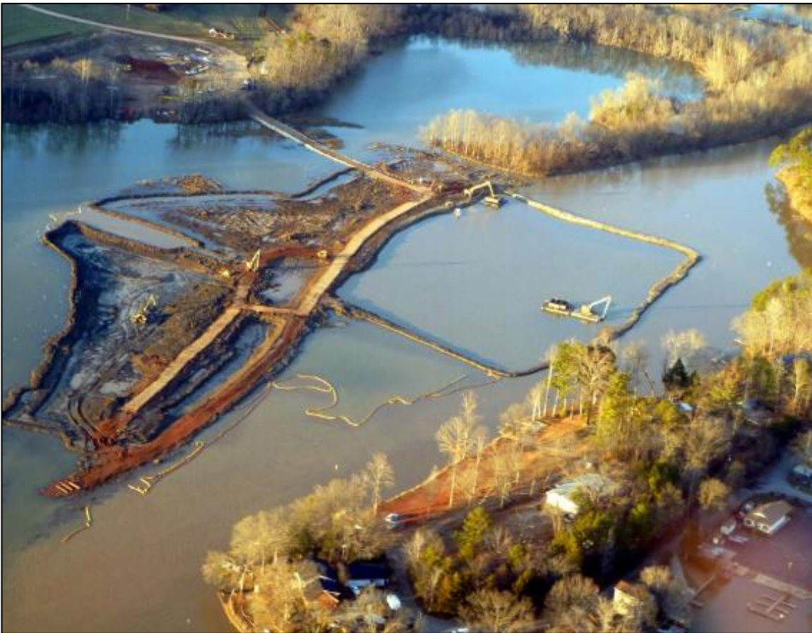
Photo 5. Saluda Lake Dredging Operation, 2012
