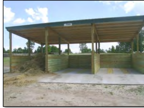
Example of Large Composter for Waste Management
