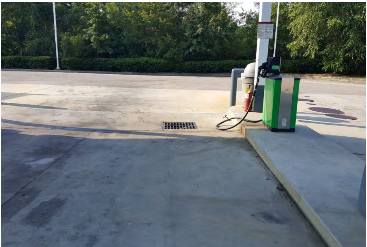
Figure 22. Gas station’s drop inlet under canopy
