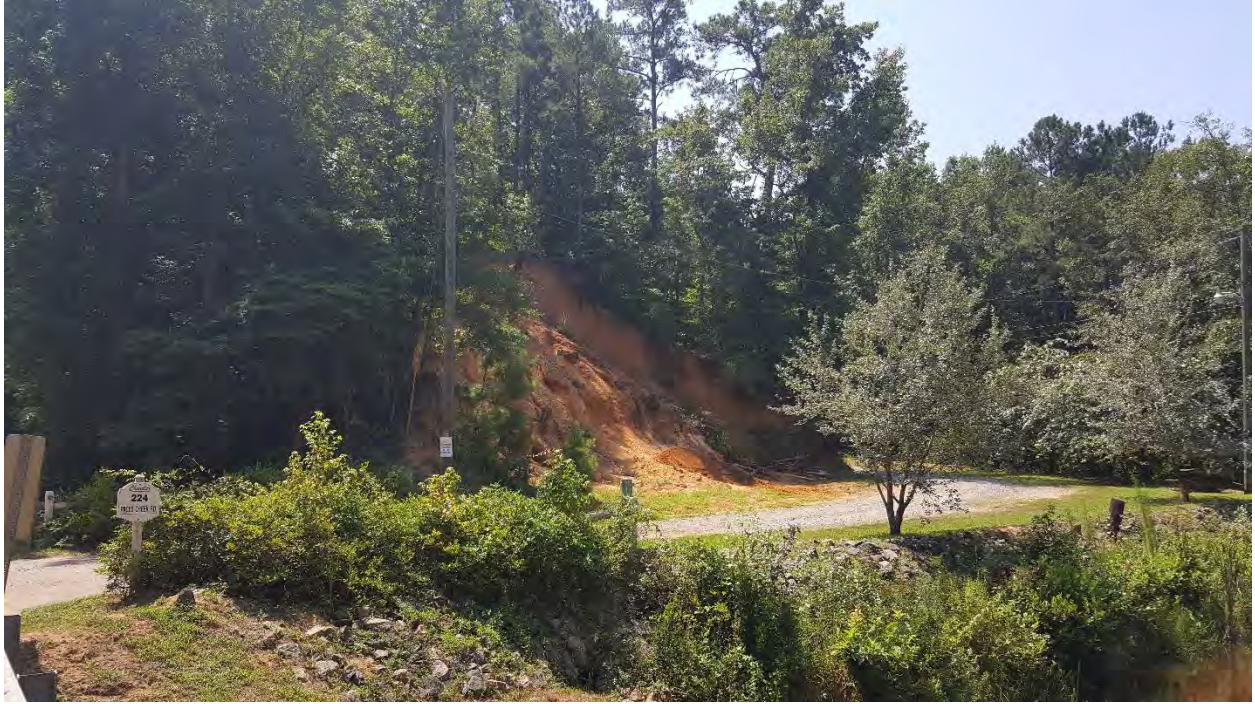
Figure 13. Unstable embankment adjacent to Paces Branch
