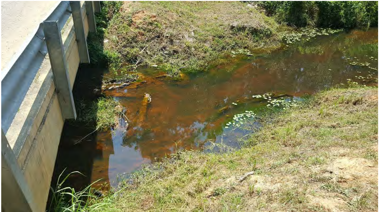
Figure 14. Observed sediment and algae in Paces Branch downstream of eroded embankment
