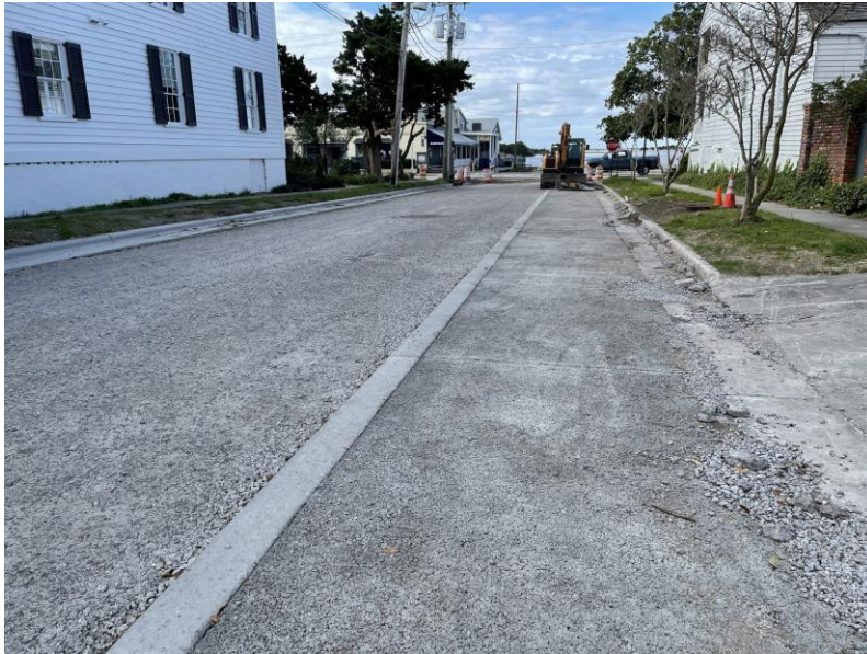
FIGURE 61: PERMEABLE PAVING INSTALLATION IN BEAUFORT, NC
