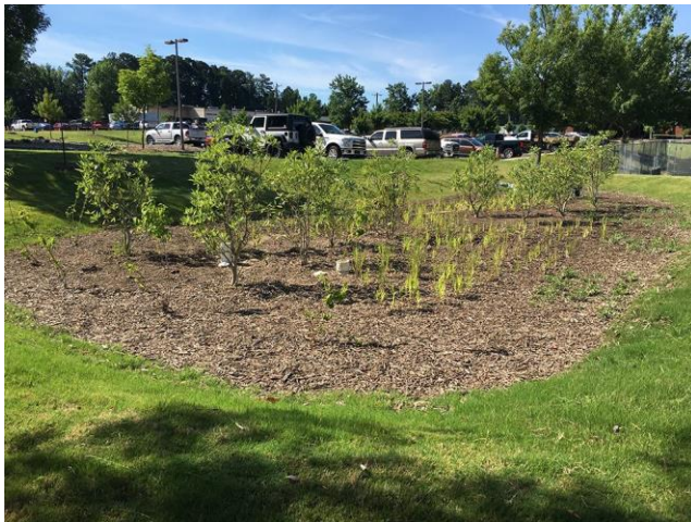
FIGURE 56. A BIORETENTION CELL IN THE CITY OF DURHAM FILTERS RUNOFF FROM THE ADJACENT PARKING LOT
