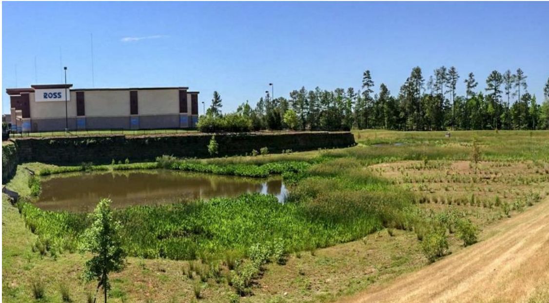
FIGURE 60: A NEWLY INSTALLED CONSTRUCTED WETLAND IN NORTH CAROLINA
