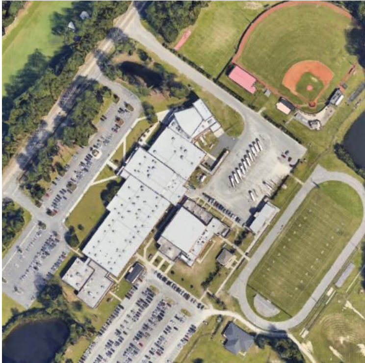
FIGURE 52: WACCAMAW HIGH SCHOOL HAS A VAST AMOUNT OF ROOFTOP AVAILABLE FOR RAINWATER HARVESTING
