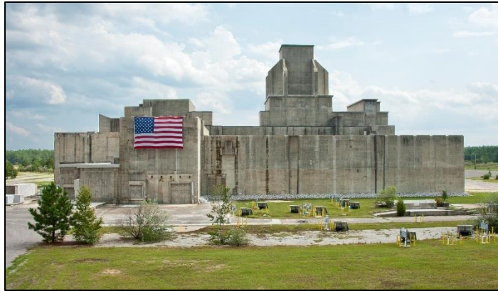
P Reactor at SRS – No longer in operation Photo by DOE-SR. CC BY 2.0
