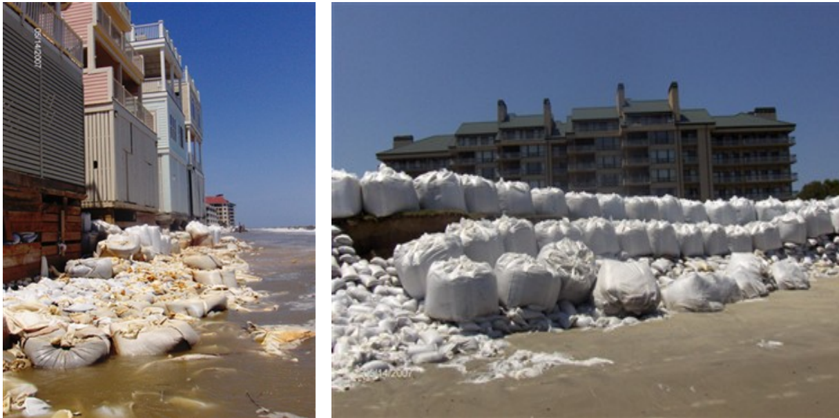
Figure 7: Five gallon and 1 cubic meter sandbags protecting structures on the Isle of Palms, SC. (2007)
