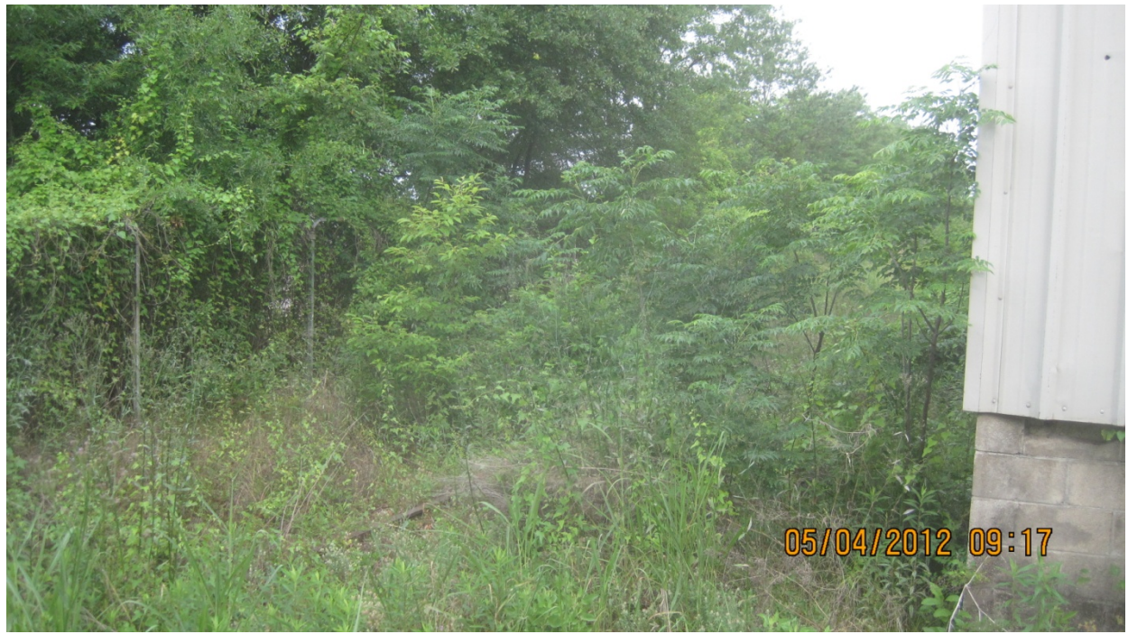
Photo 3: View of vegetated area behind warehouse building. The abandoned rail spur is hidden in the vegetation.
