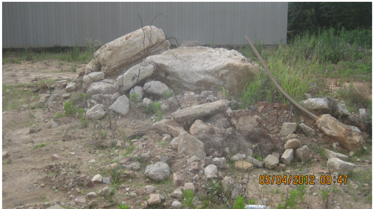
Photo 2: View of pile of construction debris in yard.
