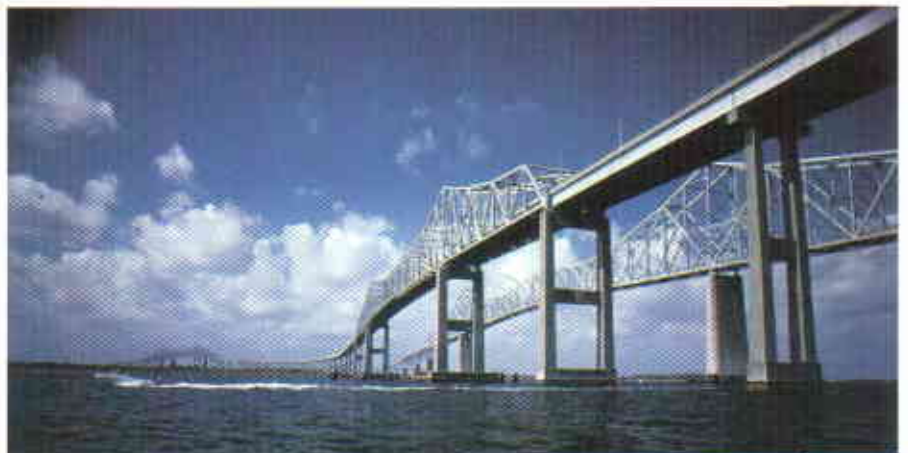
Cooper River Bridge over Charleston Harbor
