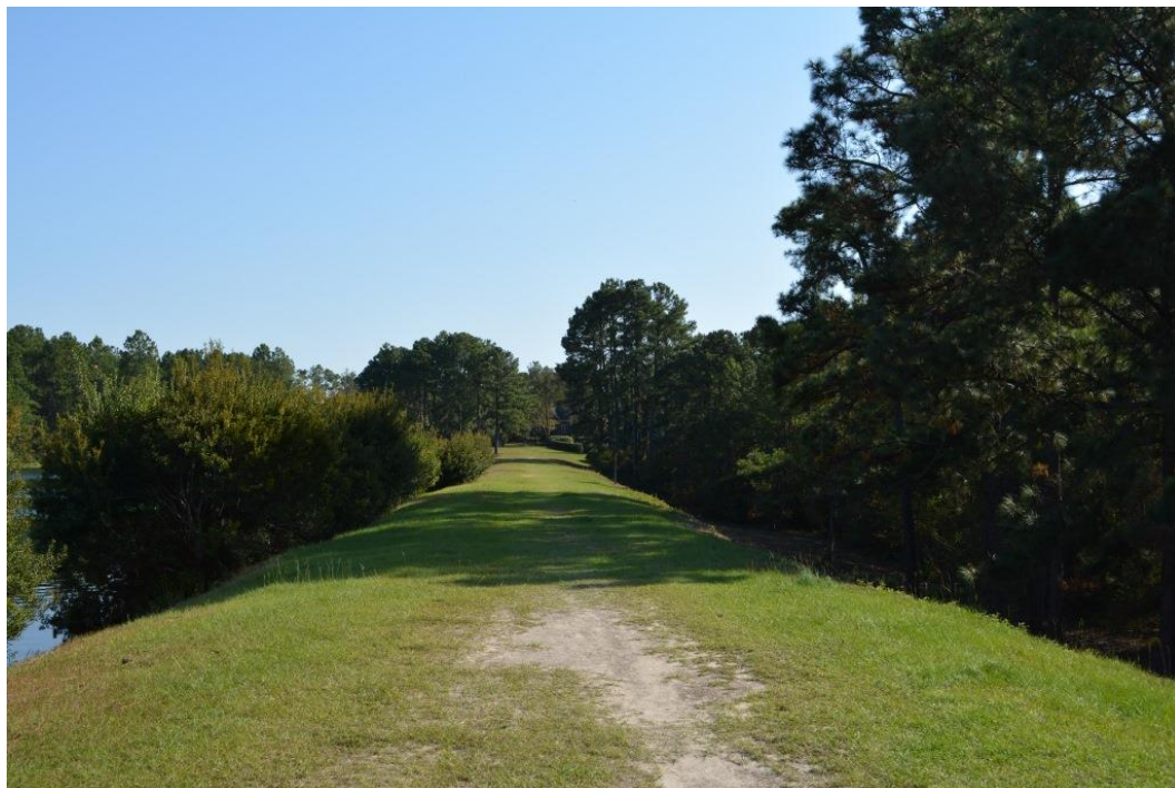
Photo 1: Embankment crest viewed from right abutment
