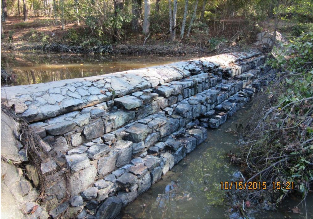
Photo 5: Auxiliary spillway upper masonry dam
