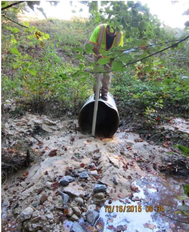
Photo 8: Service spillway outlet pipe
