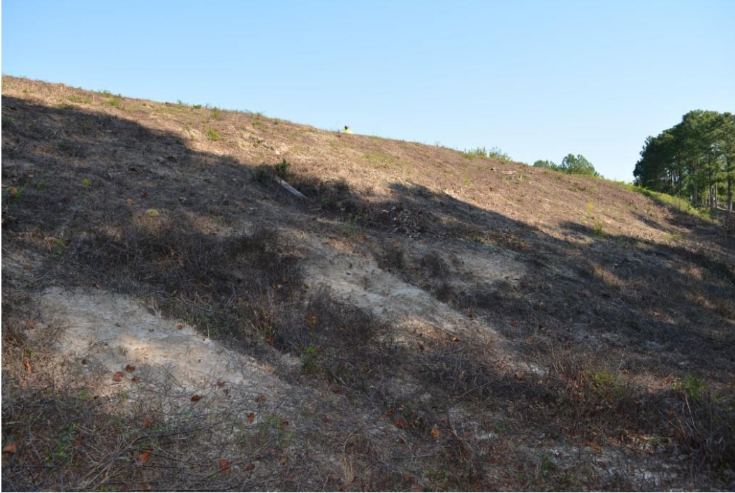
Photo 3: Downstream slope of embankment
