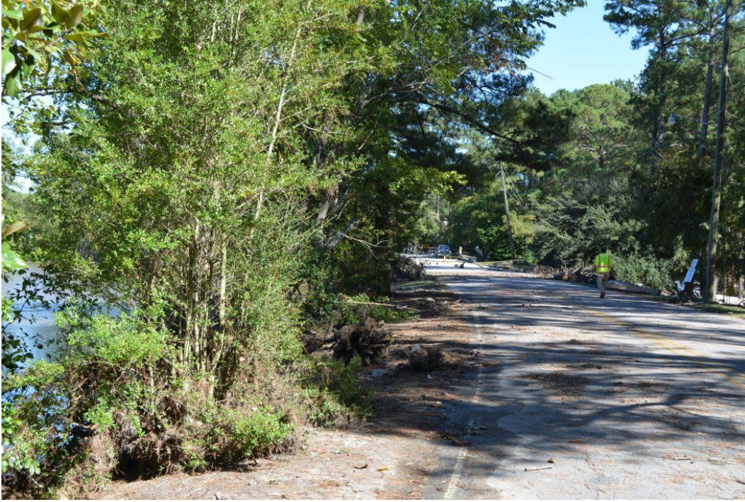
Photo 5: Crest of embankment viewed from right abutment
