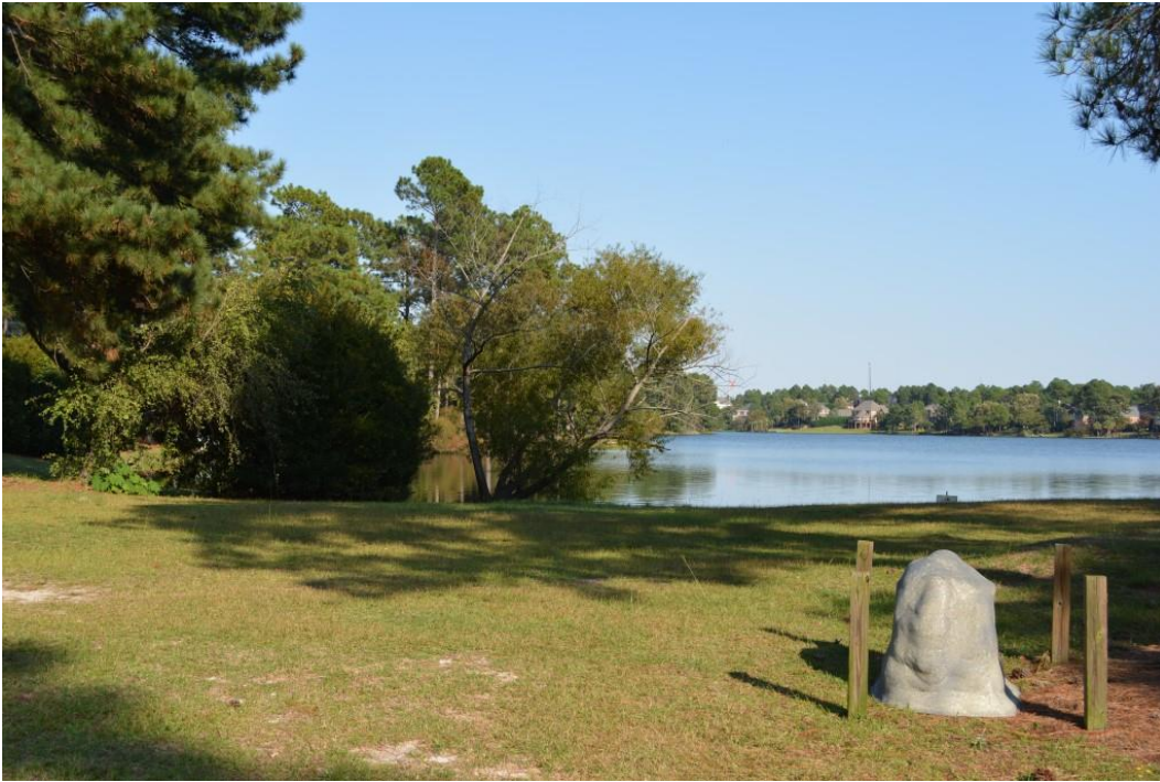
Photo 8: View of auxiliary spillway looking upstream
