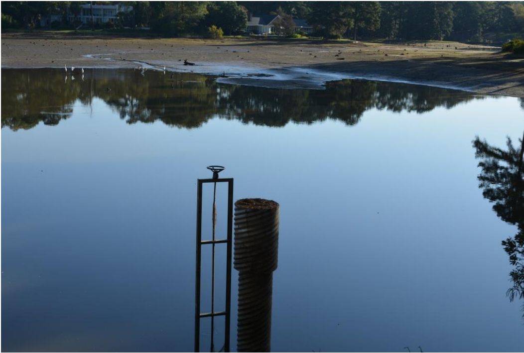
Photo 6: Service spillway intake
