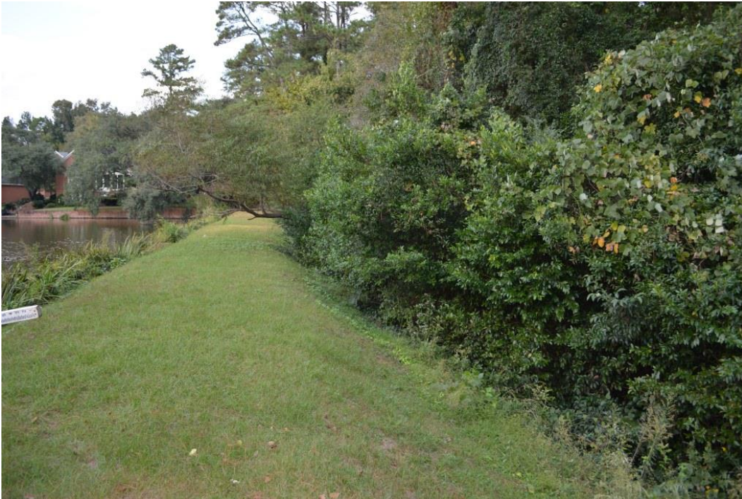
Photo 4: Downstream embankment slope
