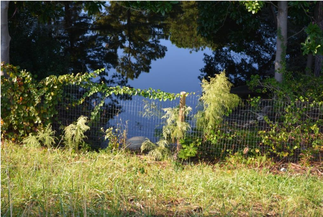
Photo 6: Tailwater and outlet pipe
