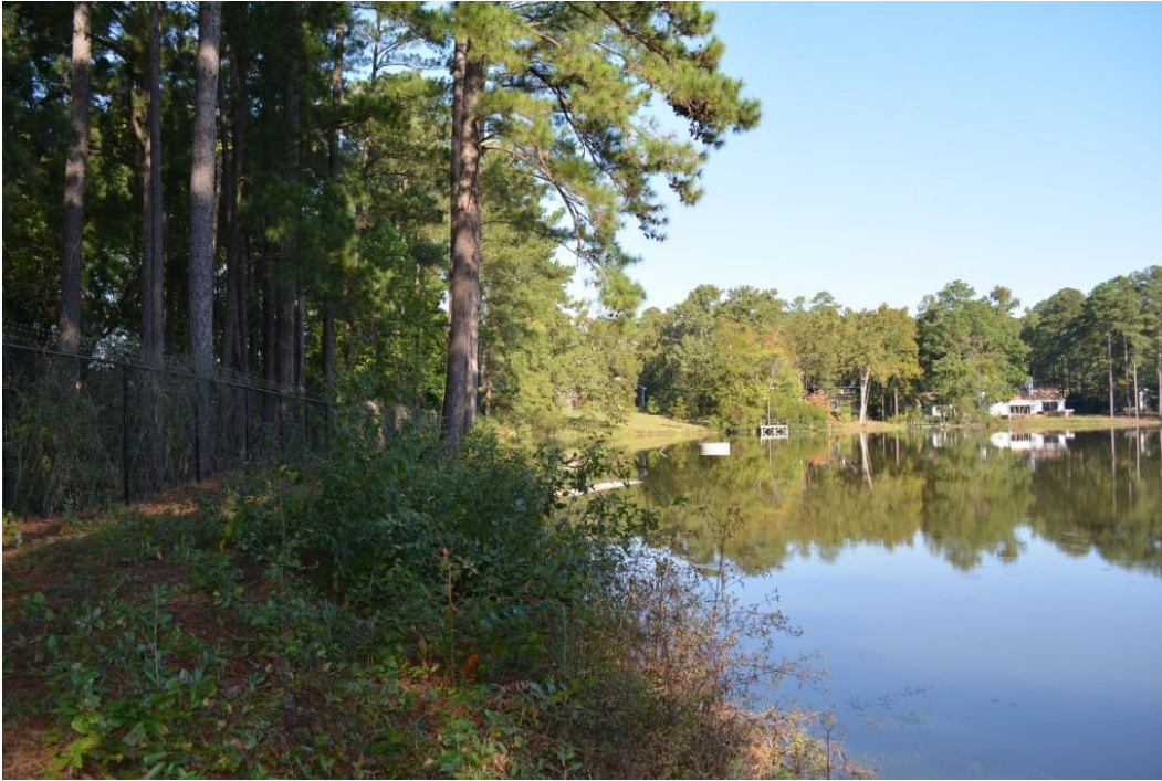
Photo 1: Lower Spring Valley Lake viewed from left abutment; the upstream embankment slope is in the foreground
