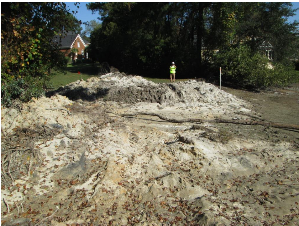
Photo 4: Temporary channel viewed from the embankment
