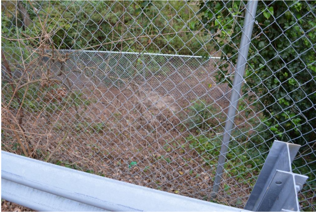
Photo 3: View of embankment downstream slope from crest
