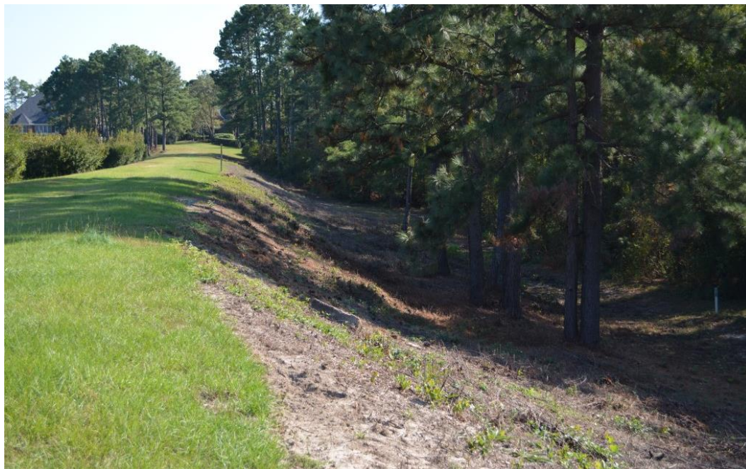
Photo 2: Downstream slope of embankment
