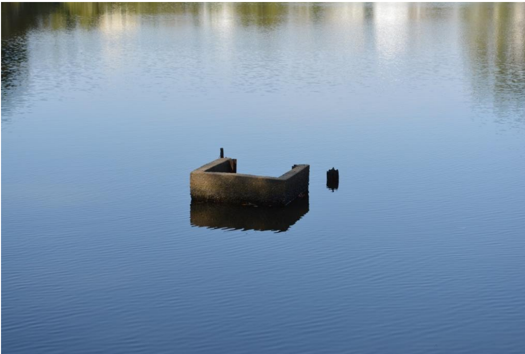
Photo 6: Intake structure (possibly abandoned)
