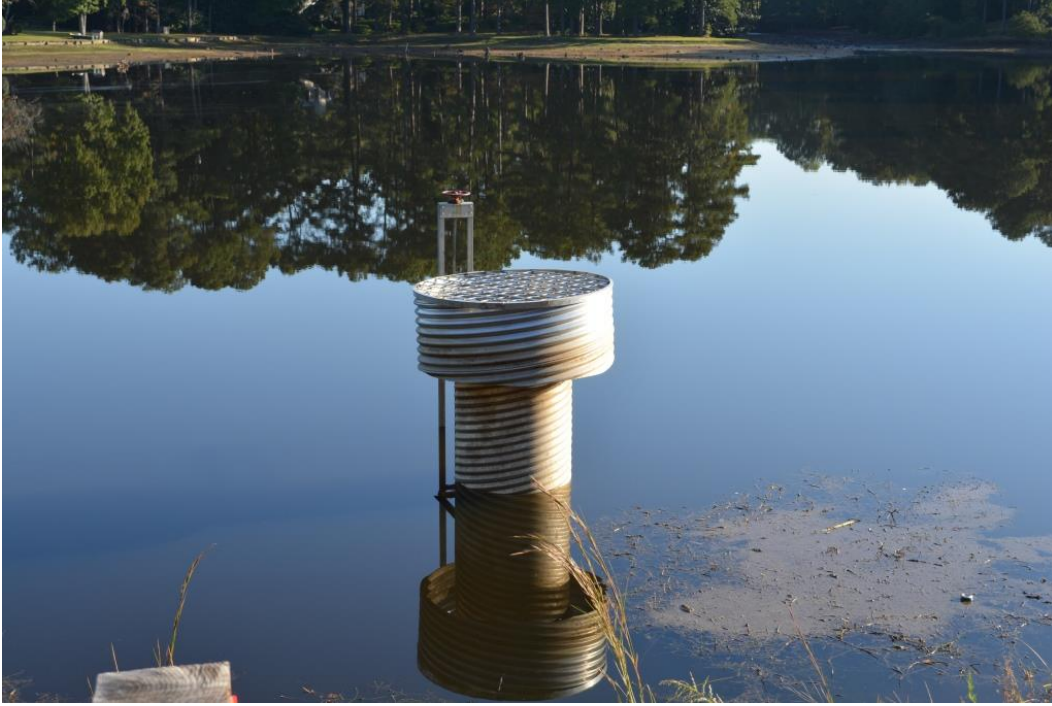
Photo 5: Service spillway intake
