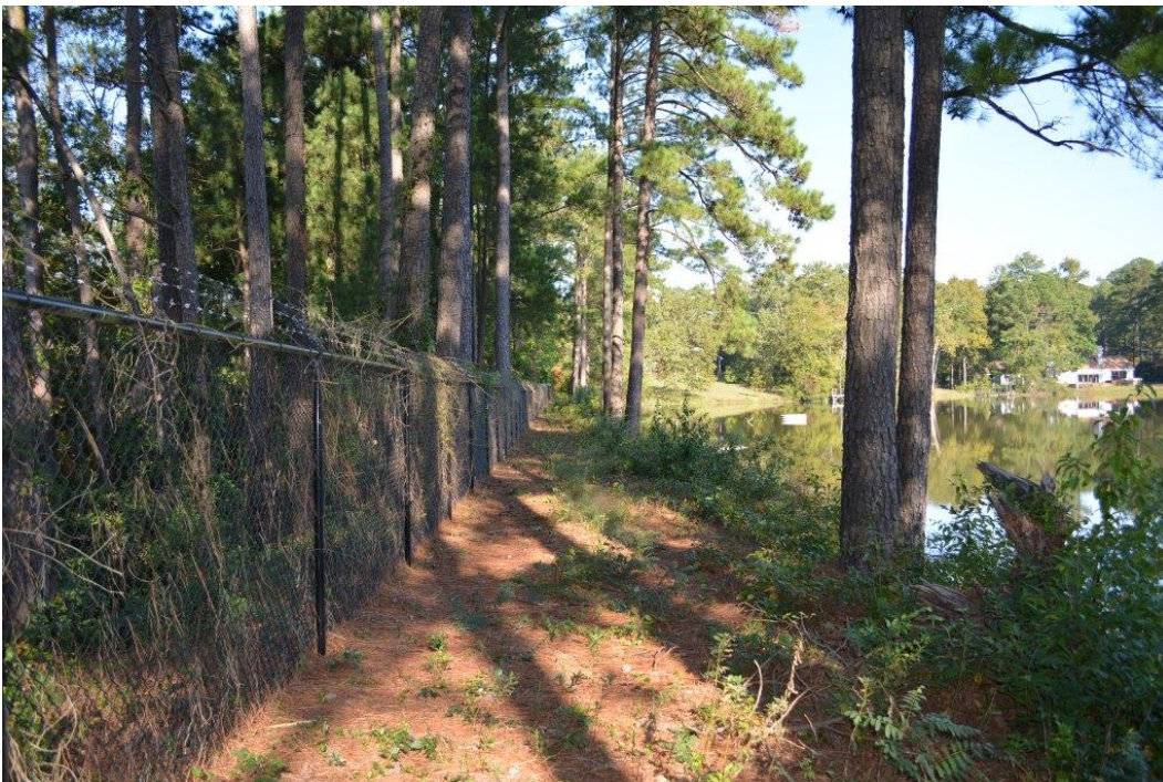
Photo 2: Embankment dam crest viewed from the left abutment
