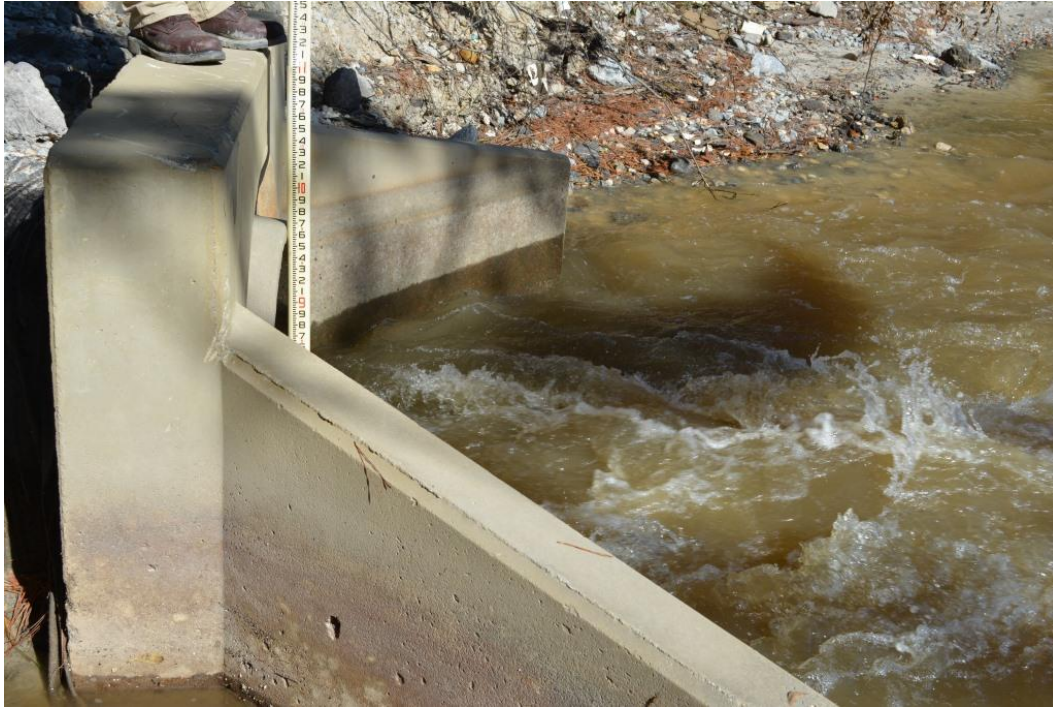
Photo 7: Service spillway outlet structure
