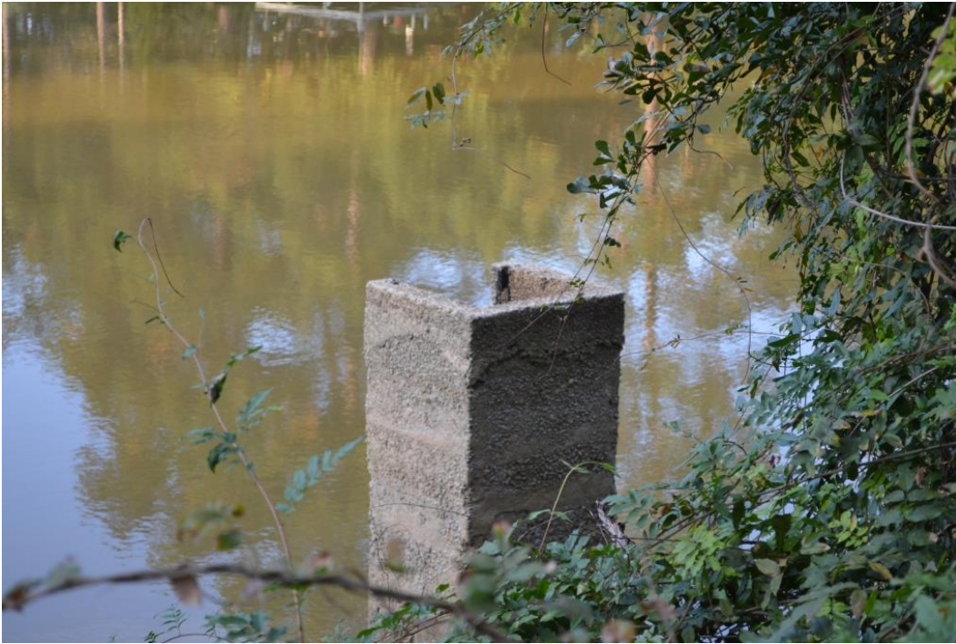
Photo 6: Service spillway drop inlet
