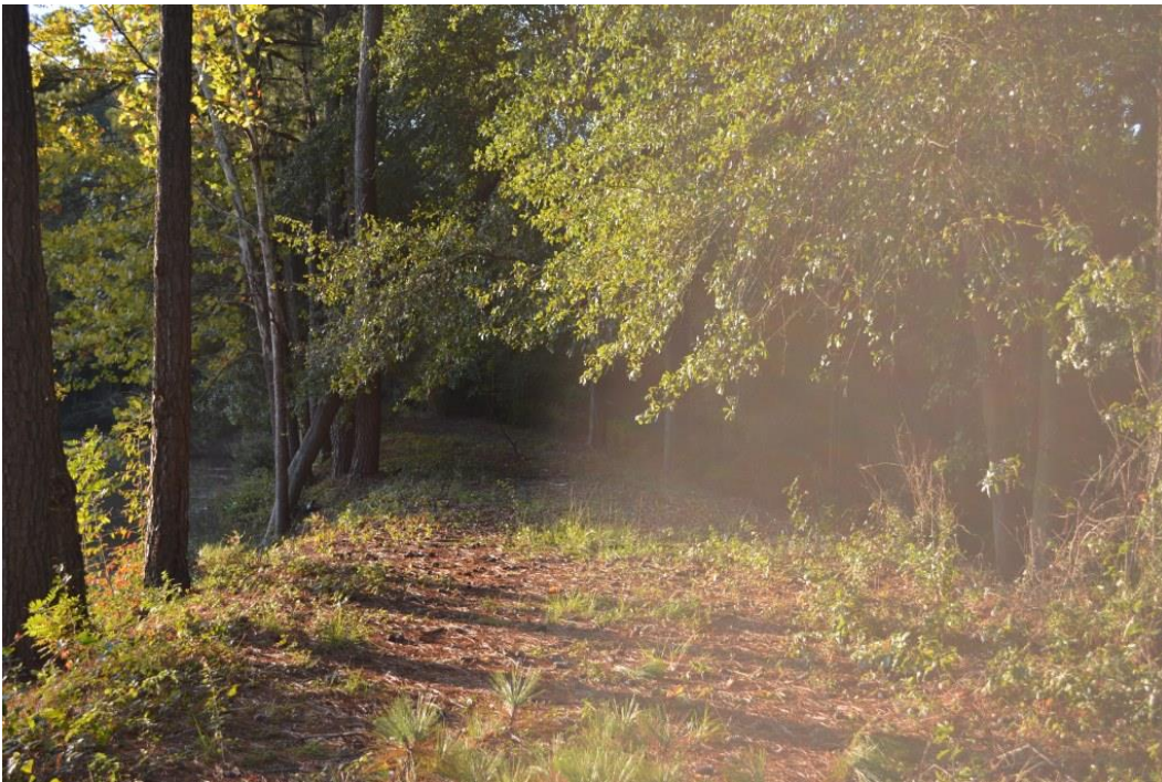
Photo 2: Embankment dam crest viewed from the right abutment
