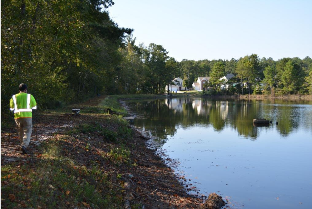
Photo 1: Deer Lake embankment dam crest and upstream slope
