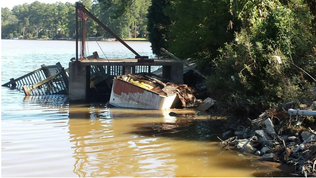
Photo 5: Concrete drop inlet at right abutment.
