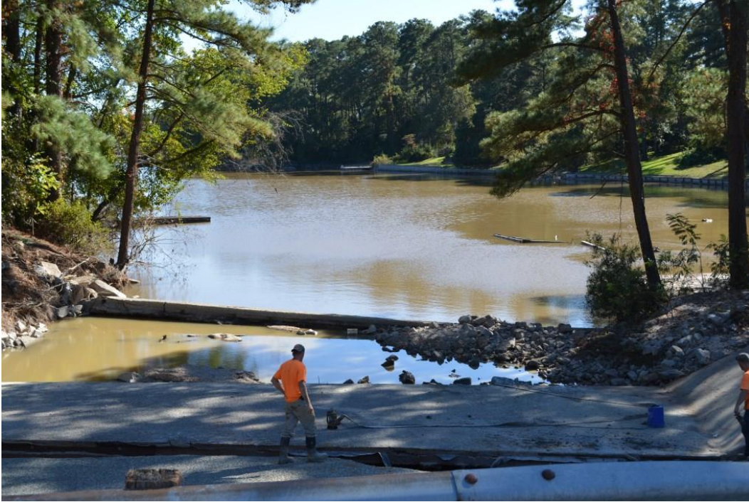
Photo 9: Downstream view from bridge over auxiliary spillway
