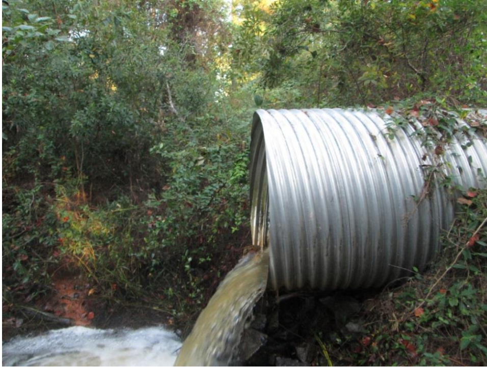
Photo 7: Service spillway outlet pipe
