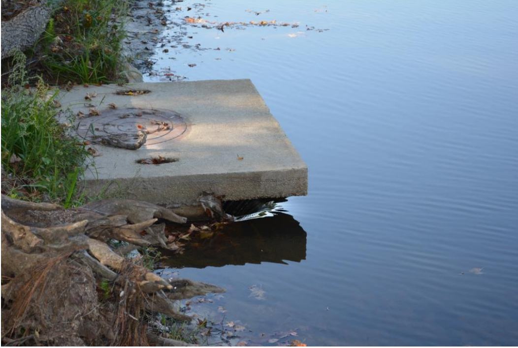
Photo 5: Service spillway intake
