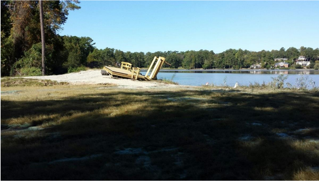
Photo 9: Auxiliary earthen spillway at left abutment looking toward left embankment
