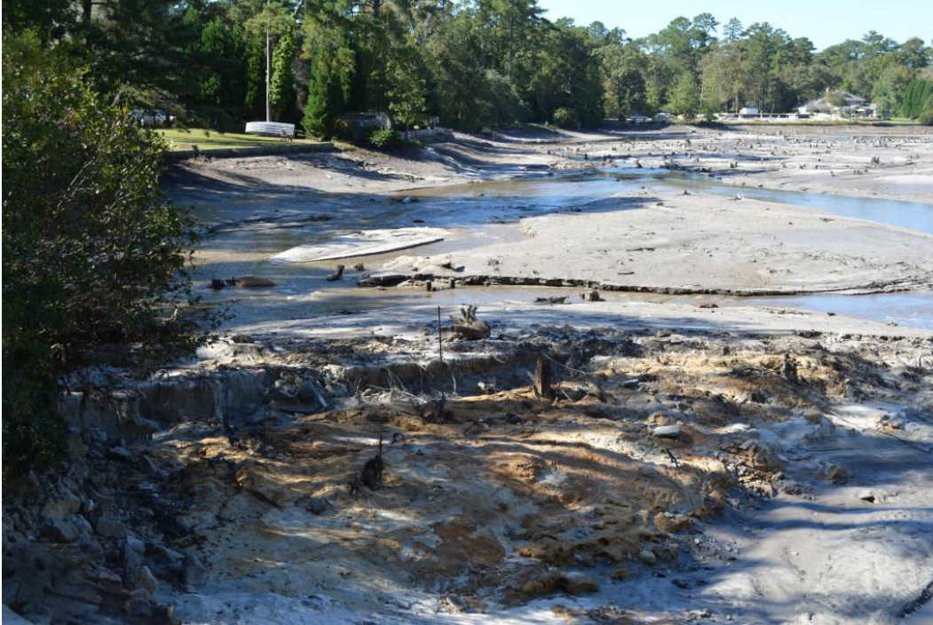
Photo 1: View upstream from the auxiliary spillway
