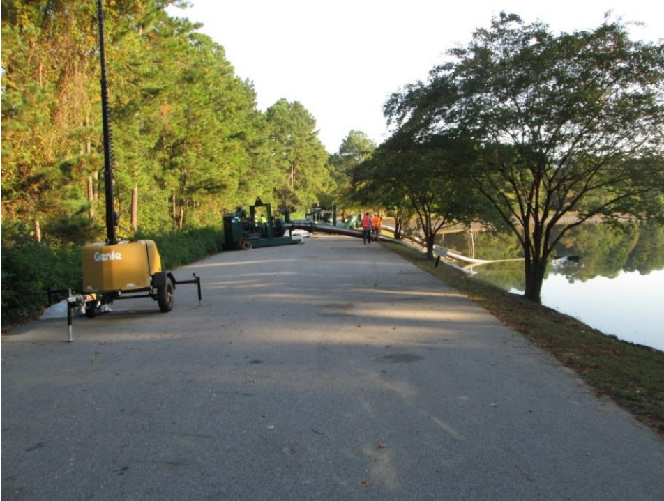
Photo 1: Embankment dam crest viewed from the left abutment.
