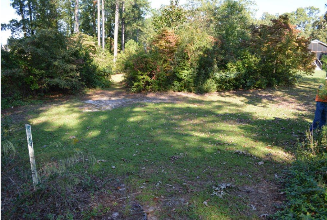
Photo 5: Auxiliary spillway at right abutment
