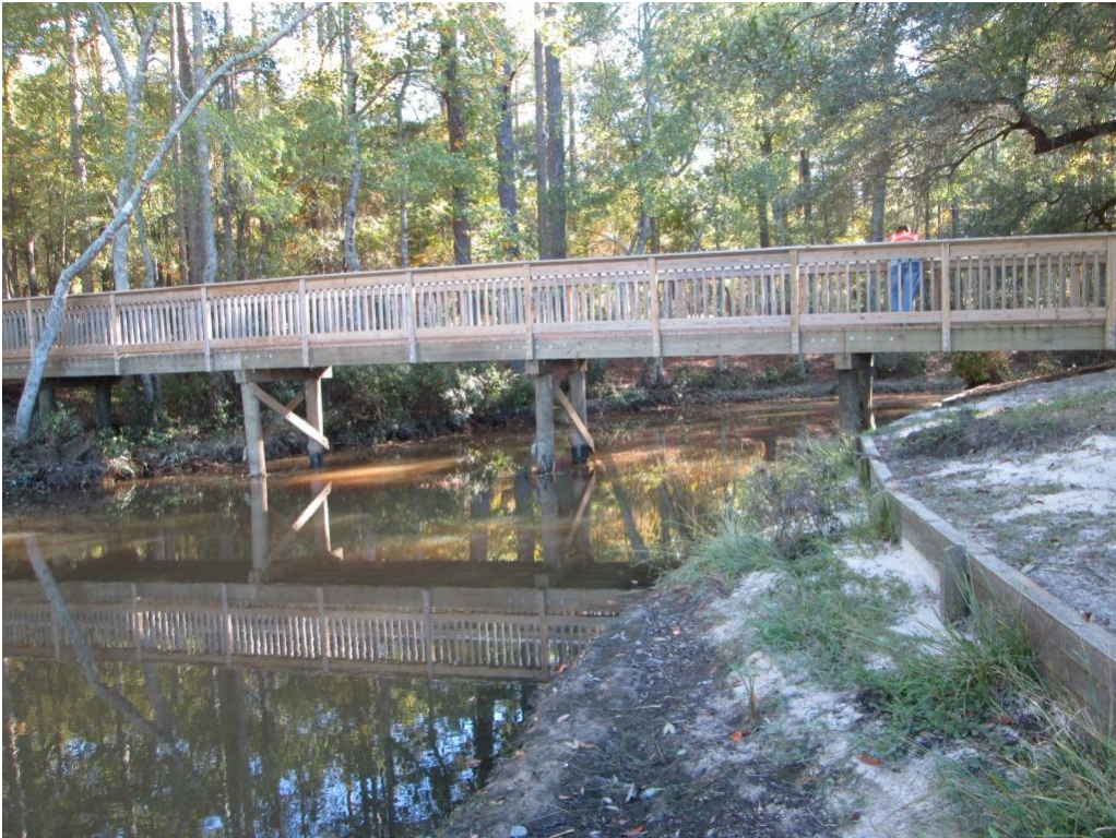
Photo 4: Approach channel to auxiliary spillway
