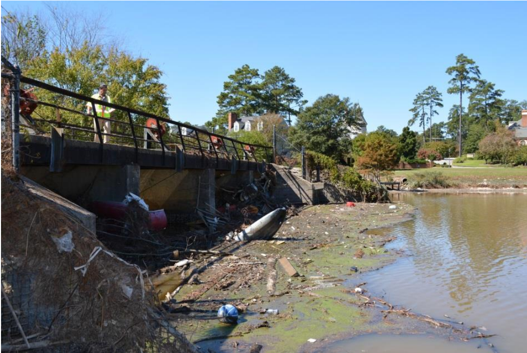
Photo 4: Upstream view of gated, concrete-buttress, overflow spillway
