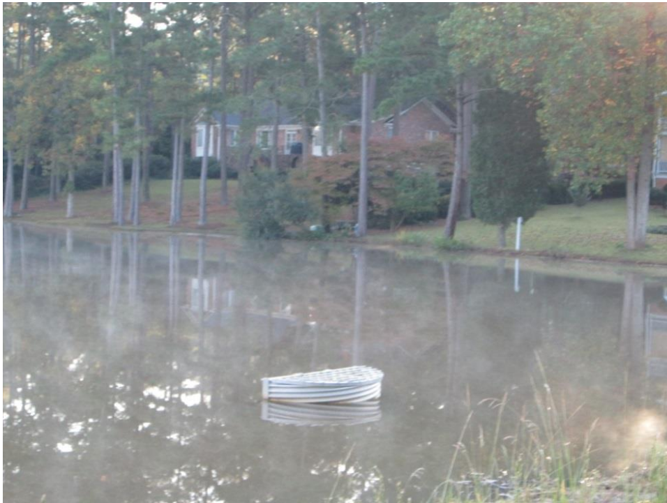
Photo 6: Service spillway inlet works.
