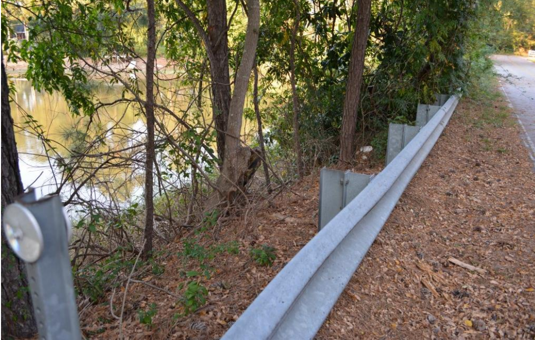
Photo 1: Upstream embankment dam slope
