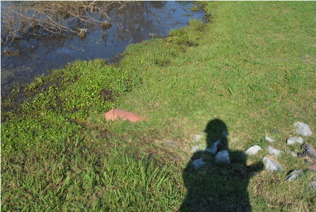
Photo 6: Auxiliary spillway looking upstream
