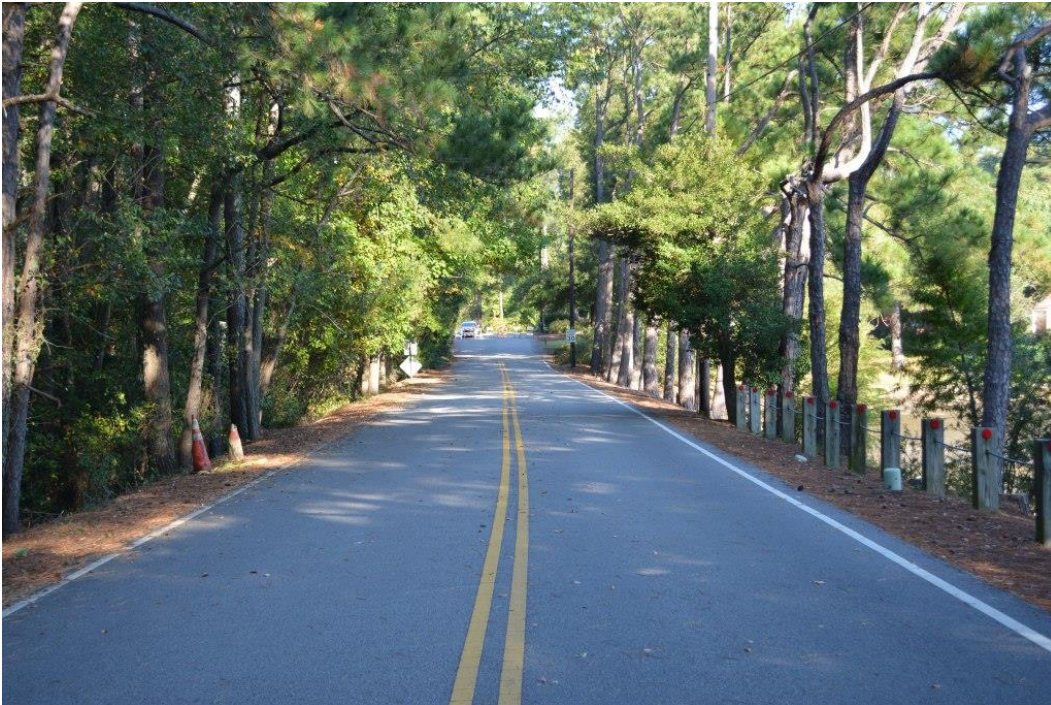
Photo 2: Roadway along embankment crest
