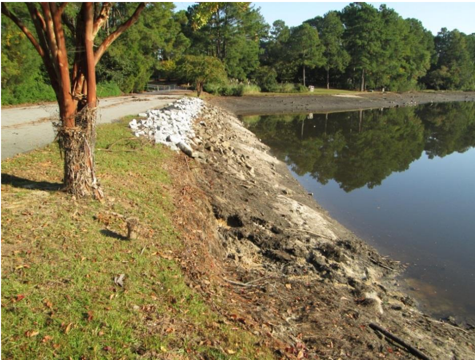
Photo 4: Temporary riprap on upstream embankment slope (looking toward the right abutment).
