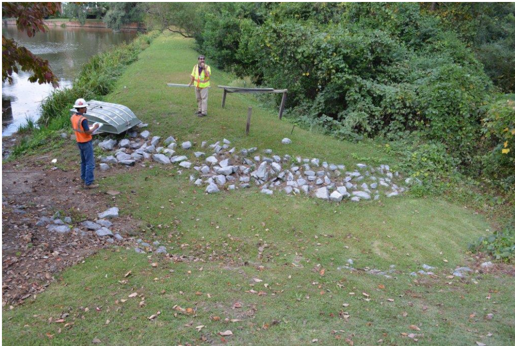
Photo 8: Commons Pond auxiliary spillway viewed from right abutment
