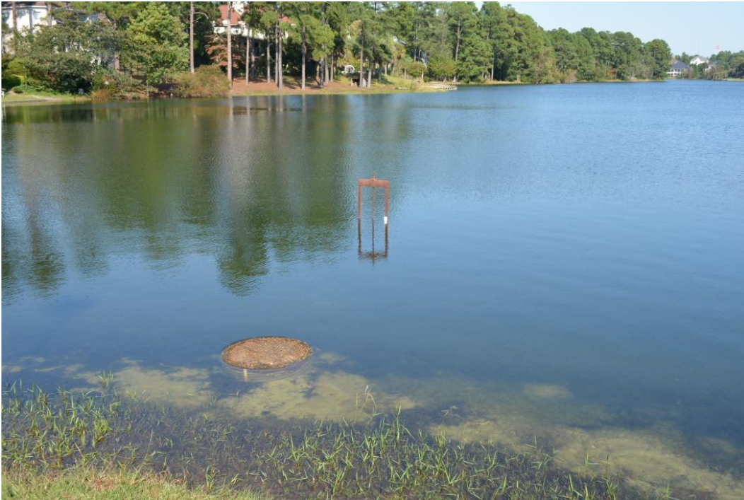
Photo 4: Service spillway intake and control
