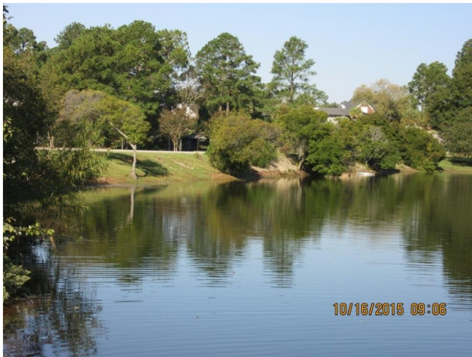
Photo 1: Embankment dam viewed from left abutment
