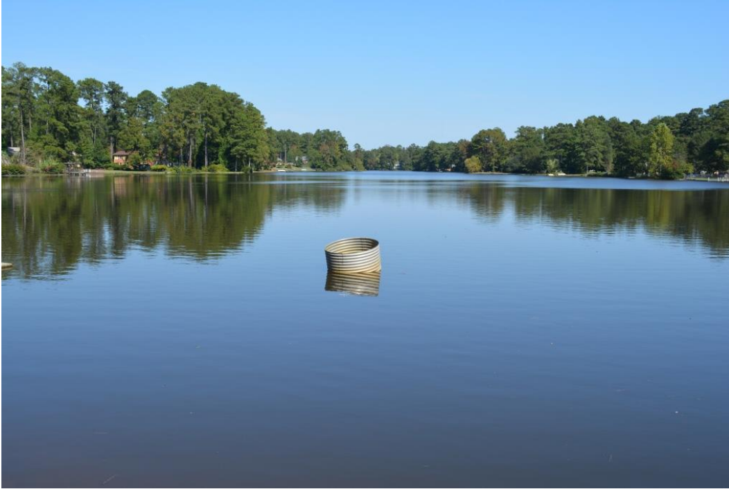
Photo 5: Service spillway intake
