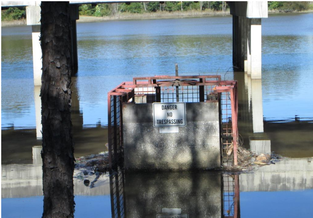
Photo 4: Service spillway drop inlet
