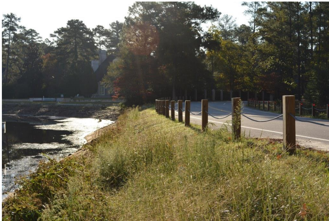
Photo 1: Upstream embankment slope
