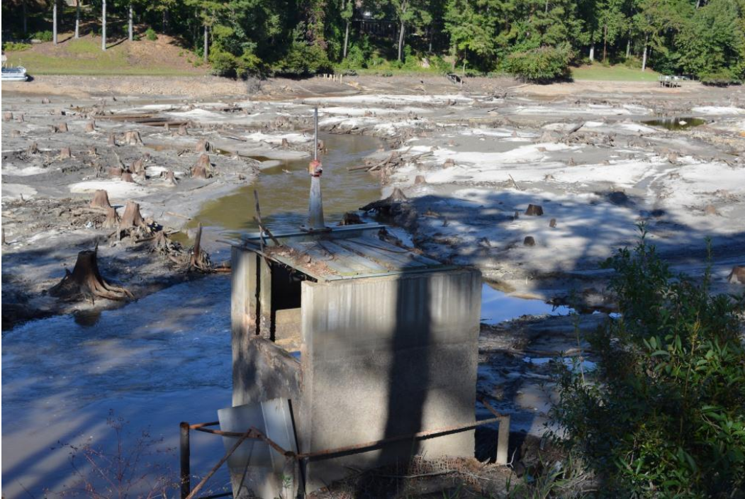
Photo 1: Service spillway drop inlet structure
