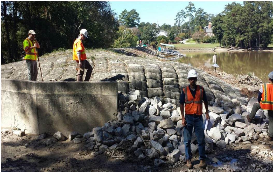
Photo 8: Temporary riprap repair upstream end of the auxiliary spillway concrete chute
