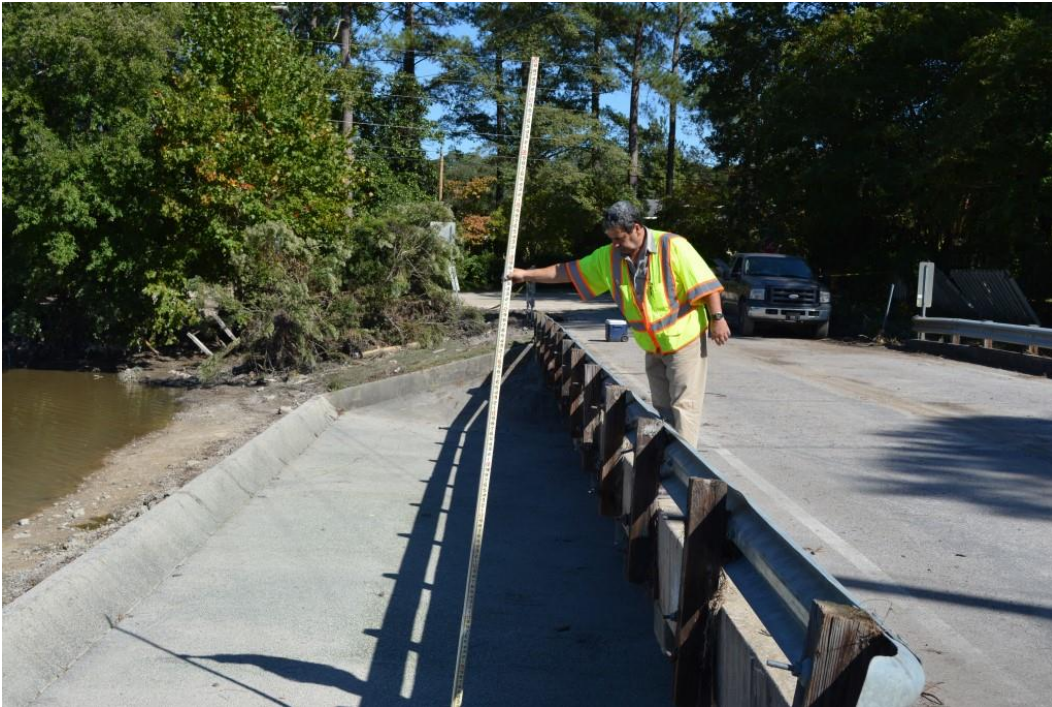
Photo 10: View of auxiliary spillway upstream of bridge
