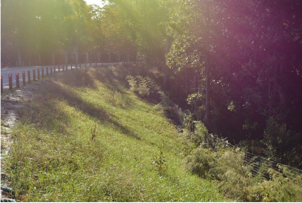
Photo 3: Downstream embankment slope
