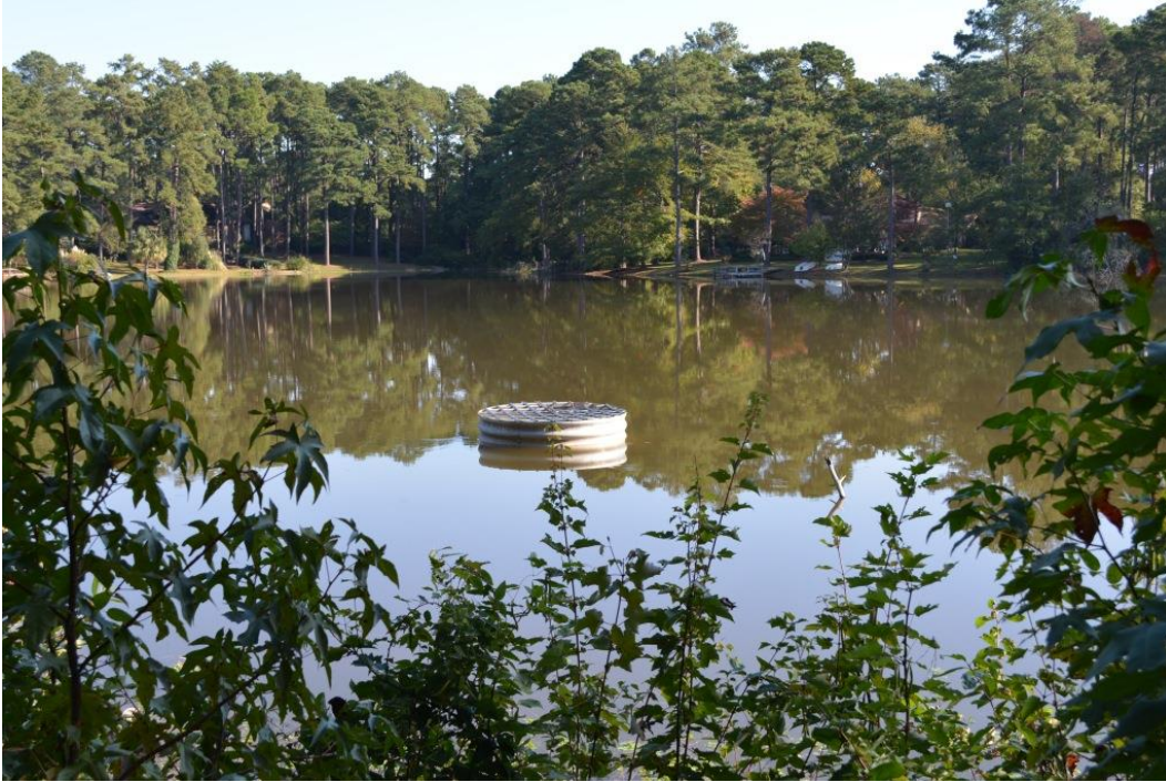
Photo 3: Service spillway intake
