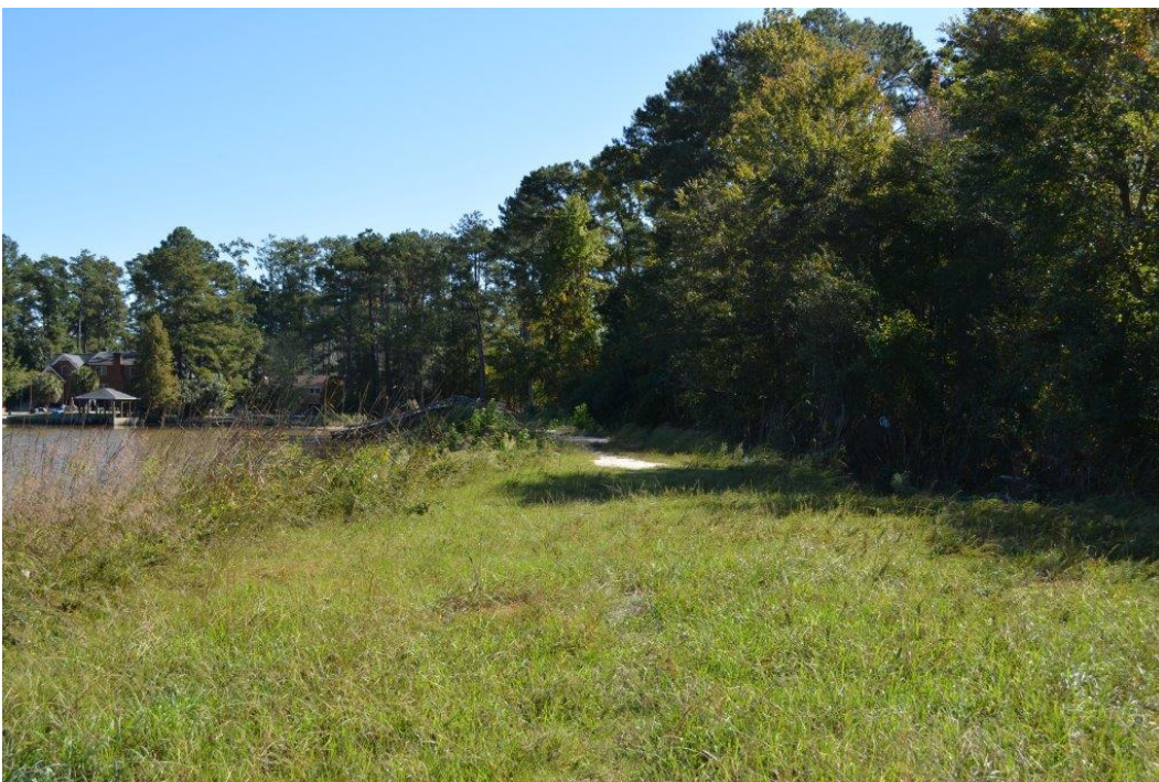
Photo 2: View of left embankment crest looking toward left abutment.
