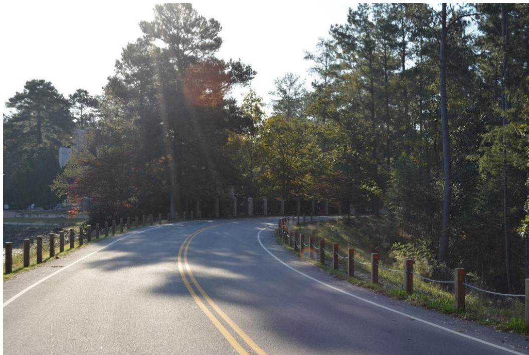
Photo 2: Roadway on embankment crest
