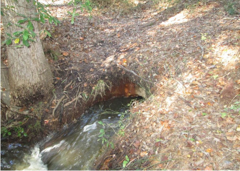
Photo 3: Service spillway outlet works
