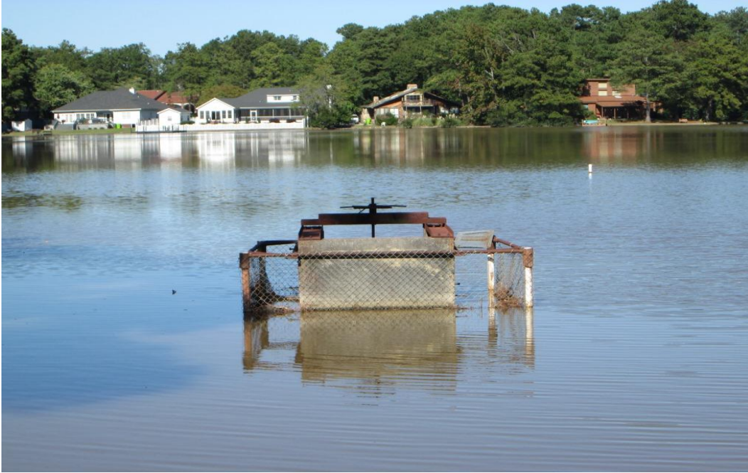
Photo 9: Service spillway drop inlet structure
