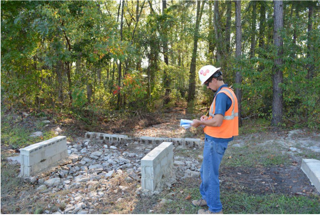
Photo 8: Auxiliary spillway view looking downstream
