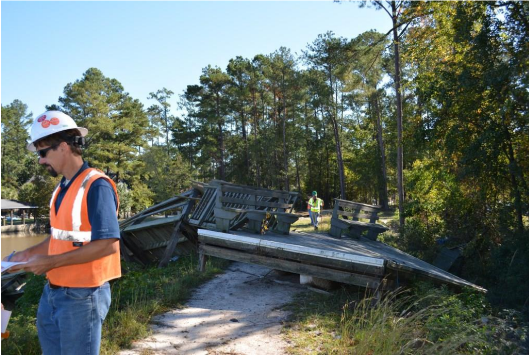
Photo 1: Dock remnants on left embankment crest
