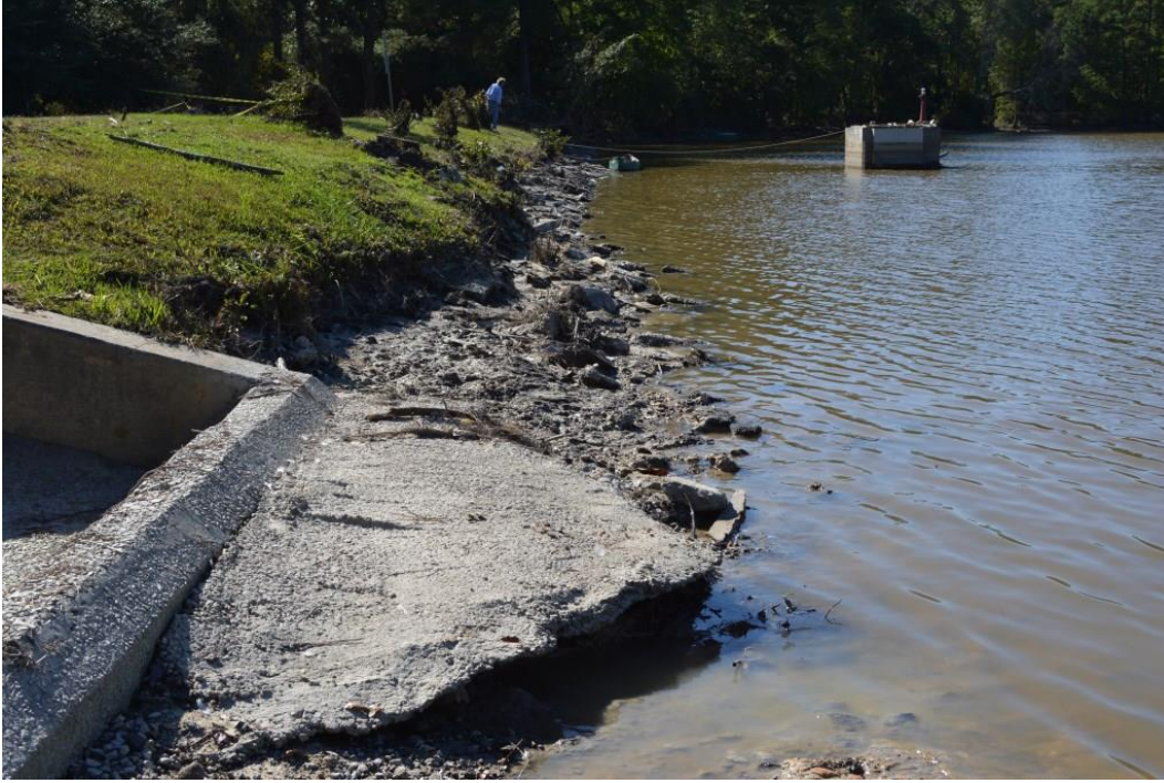
Photo 3: View of upstream embankment slope from auxiliary spillway
