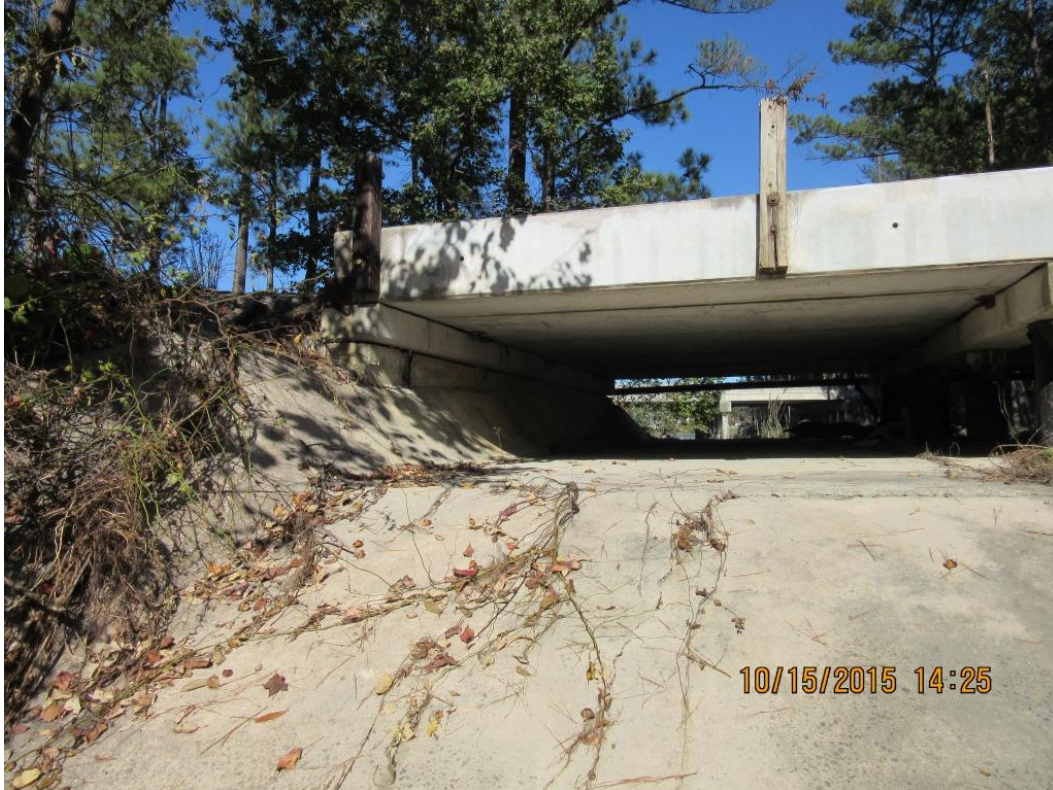
Photo 5: Auxiliary spillway viewed from the downstream side
