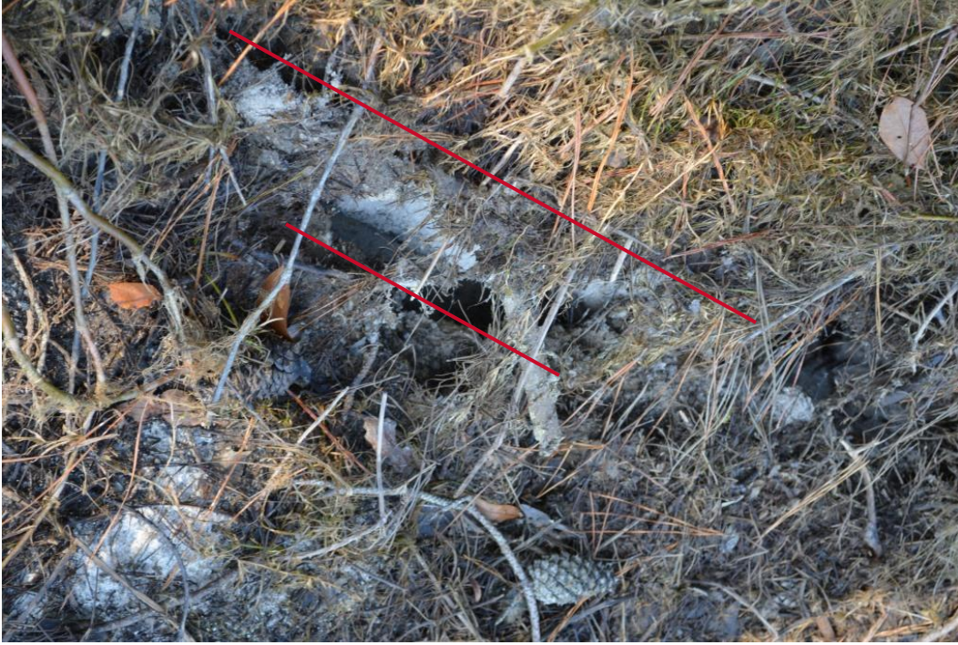
Photo 5: Longitudinal cracks in upstream embankment slope indicated with red lines
