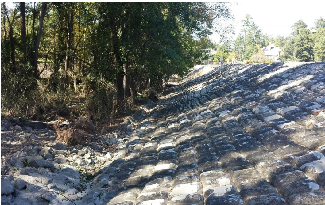
Photo 2: View along toe of the left embankment
