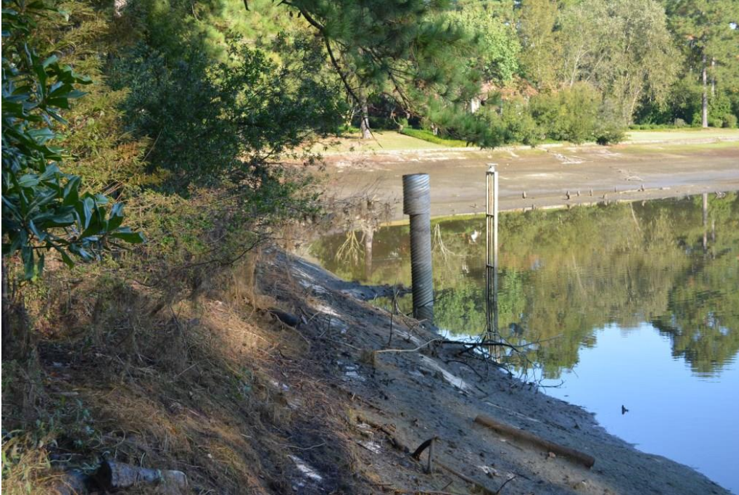
Photo 1: Upstream slope and service spillway intake
