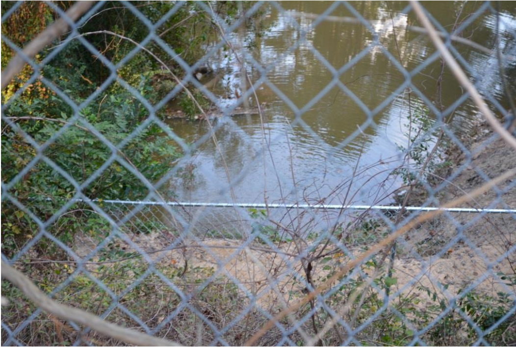
Photo 7: Service spillway outlet
