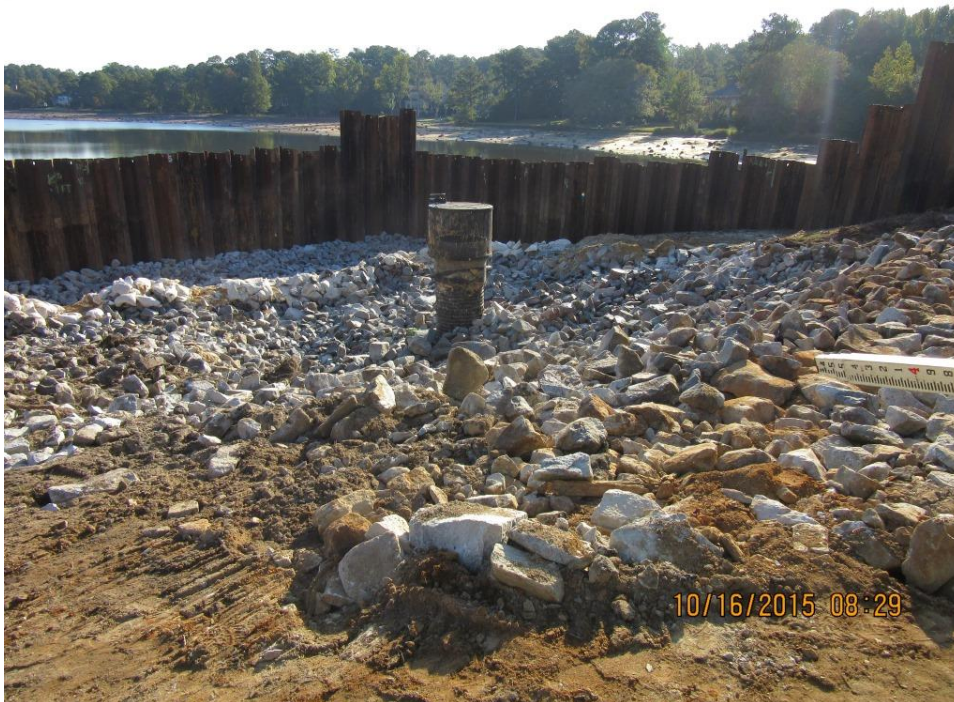
Photo 4: Rock fill placed in sinkhole area of upstream embankment slope; service spillway riser is in the foreground
