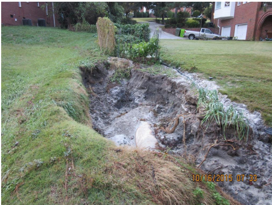
Photo 10: Eroded area at downstream end of auxiliary exposing RCP pipe, presumably a stormwater main
