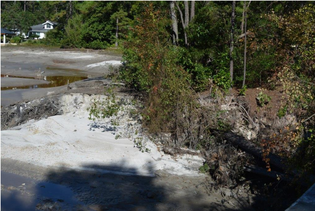
Photo 2: Erosion along the left side of approach channel to the auxiliary spillway
