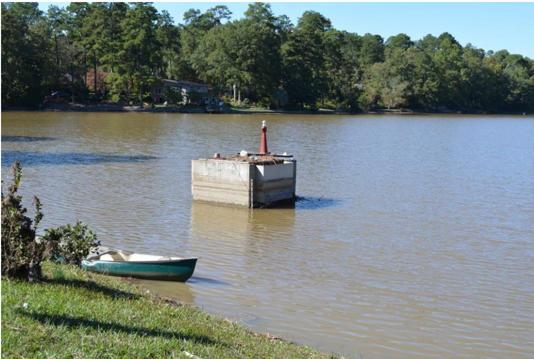
Photo 6: Service spillway drop inlet
