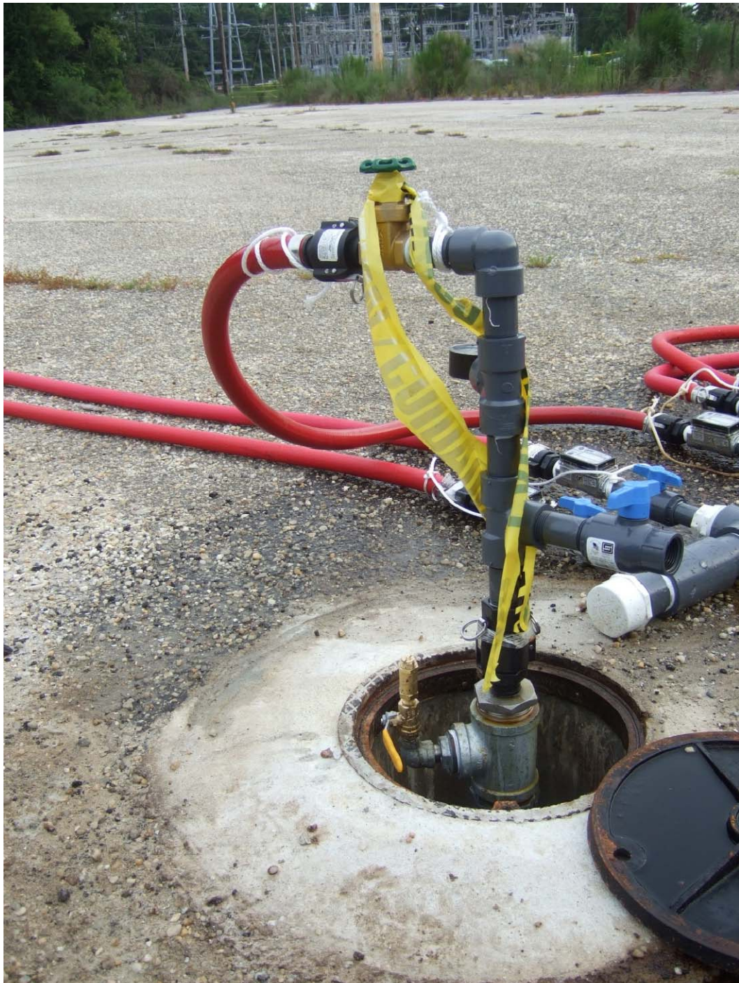
Photo #2: Typical well head apparatus with pressure relief valve.
