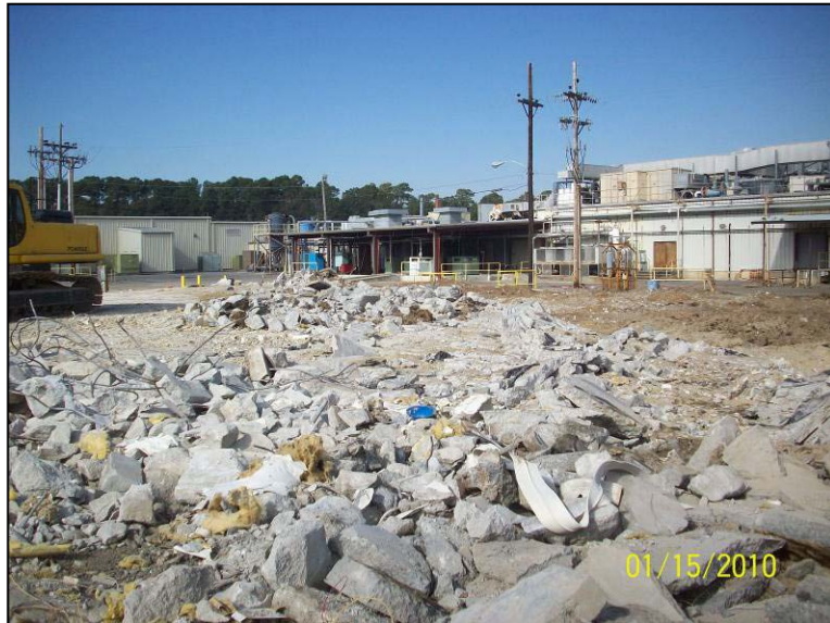
Removal of PDG Building concrete slab
