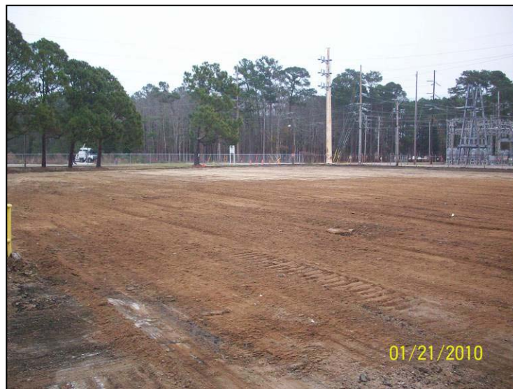
Former PDG Building location, following concrete slab removal
