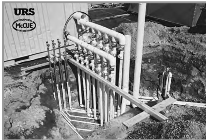
Photograph 1: AS & SVE manifolds under construction.
