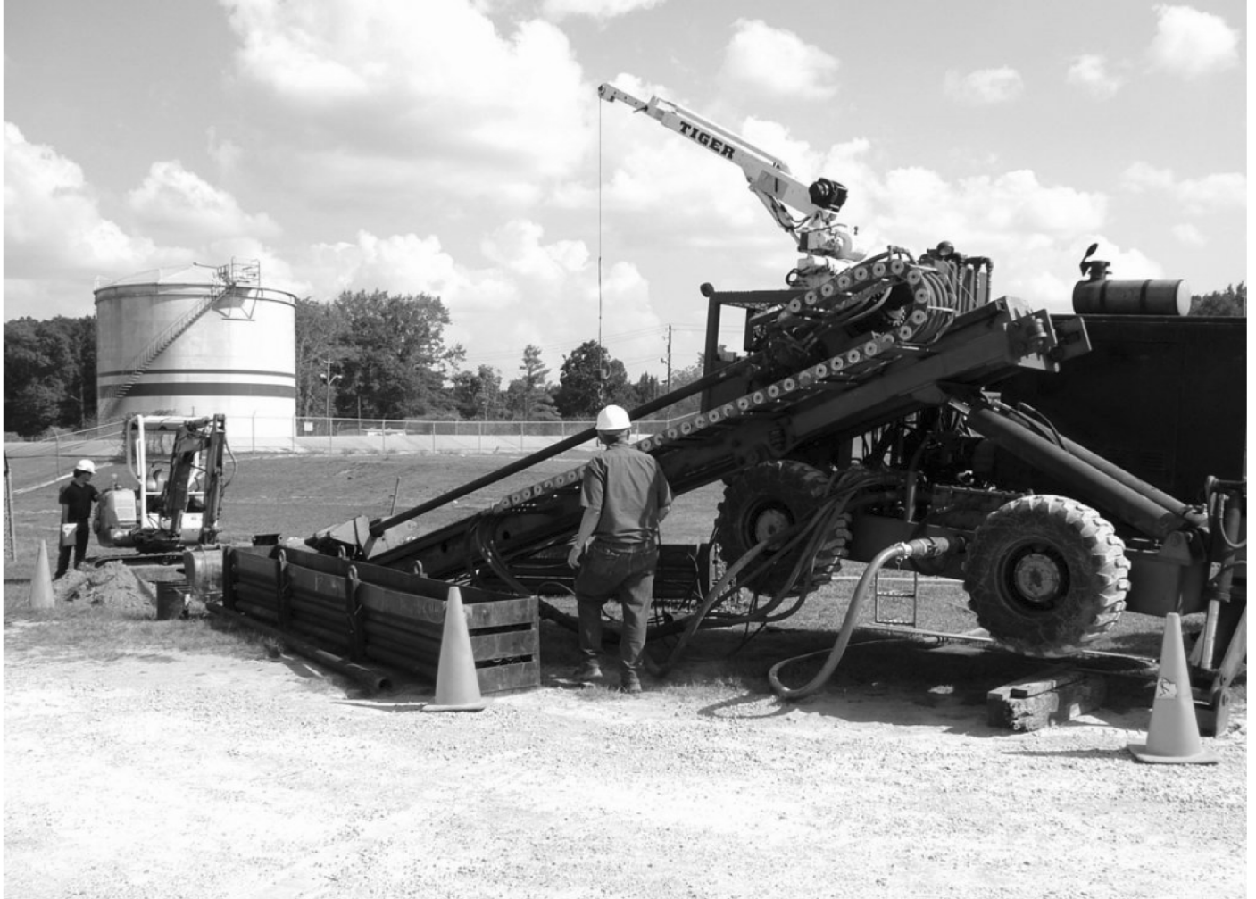
FIGURE 5. HDD well installation (Tank No. 3 in background) at Site SS-26.
