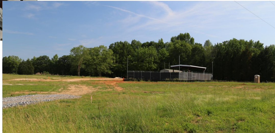
Biosparge Control Building- Street View
