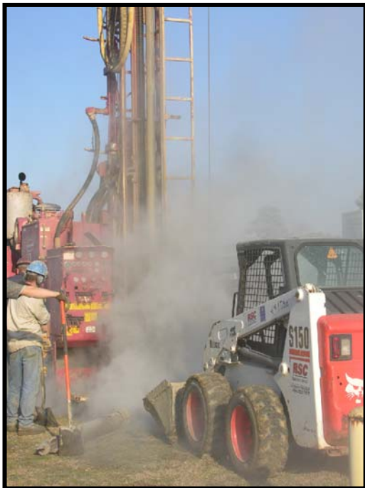
Drilling RIMW13 6 of 15
