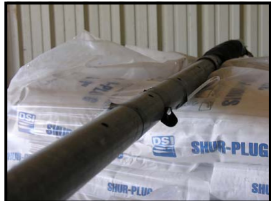
Water intakes on 10' packer assembly
