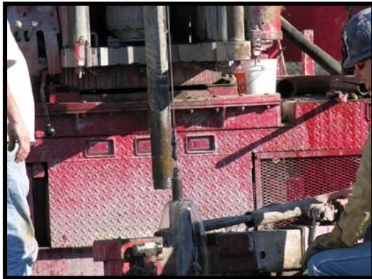
Drill rig operations 1 of 2
