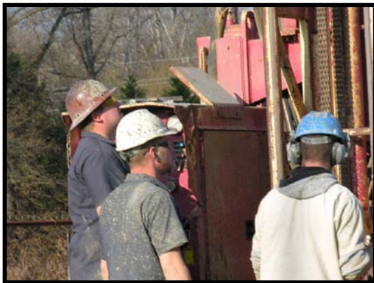
Drilling RIMW13 10 of 15
