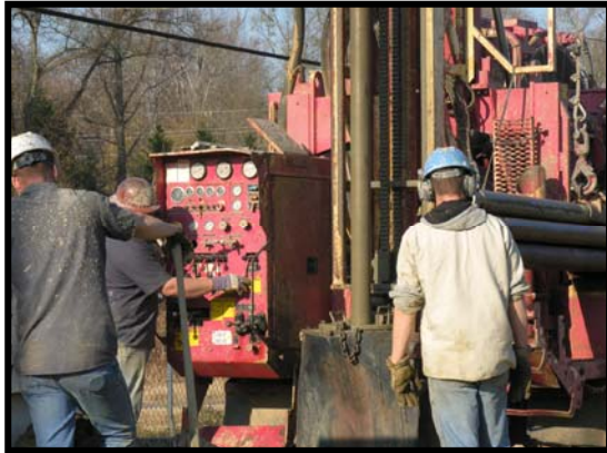
Drilling RIMW13 8 of 15
