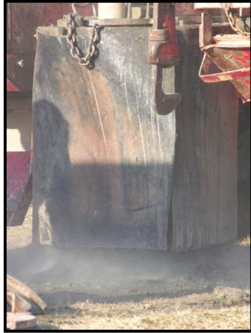
Drilling RIMW13 5 of 15
