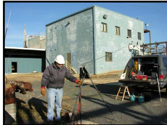
Borehole logging 2 of 2
