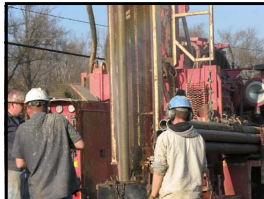
Drilling RIMW13 13 of 15
