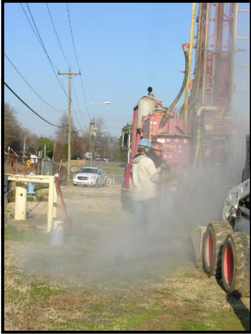
Drilling RIMW13 4 of 15
