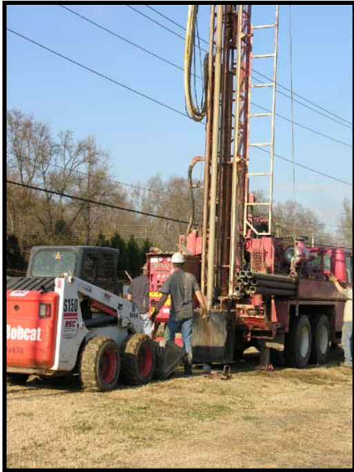
Drilling RIMW13 14 of 15
