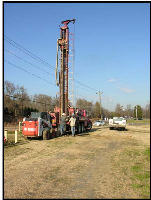
Drilling RIMW13 15 of 15
