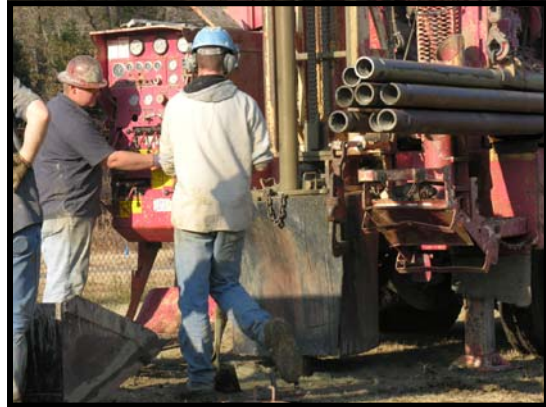
Drilling RIMW13 9 of 15
