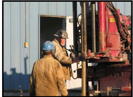
Drill rig at RIMW19 4 of 4
