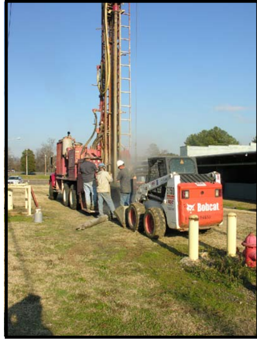
Drilling RIMW13 1 of 15
