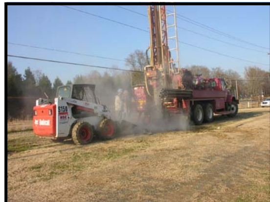
Drilling RIMW13 11 of 15
