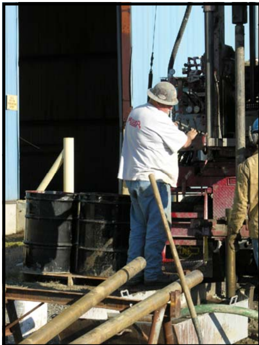
Drill rig at RIMW19 1 of 4
