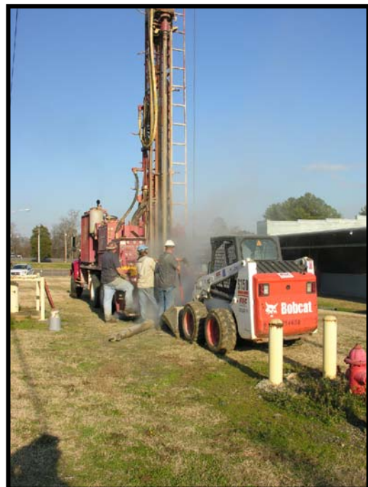
Drilling RIMW13 7 of 15
