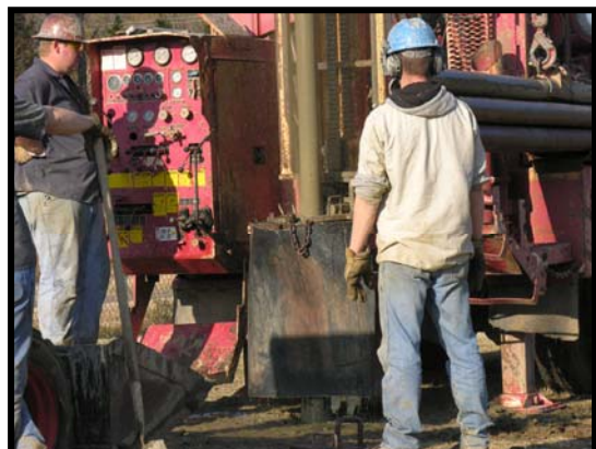
Drilling RIMW13 12 of 15
