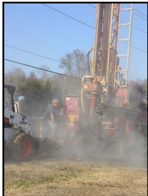
Drilling RIMW13 3 of 15
