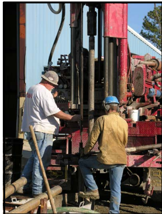
Drilling RIMW19 2 of 4
