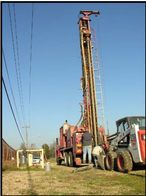
Drilling RIMW13 2 of 15
