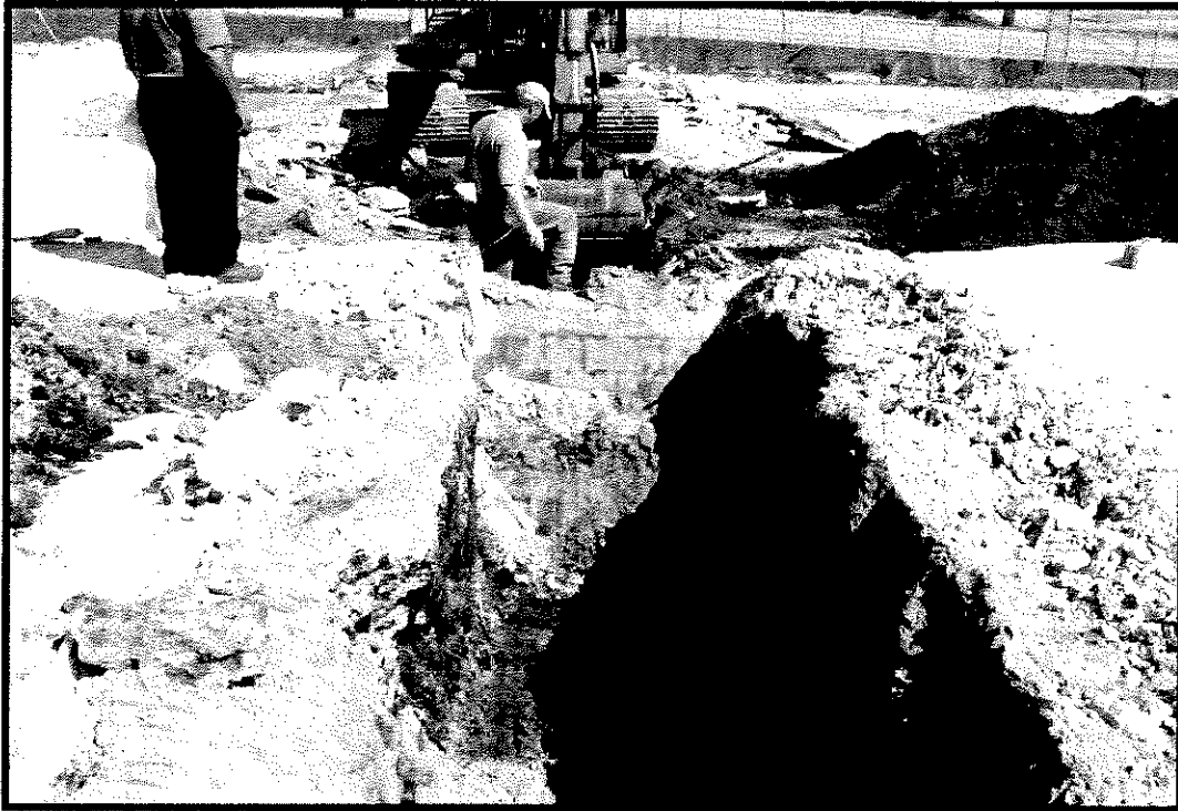
Western portion of SDTP-2 showing buried gas holder base
