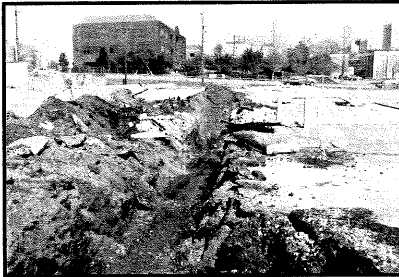
SDTP-3 central portion showing buried structure
