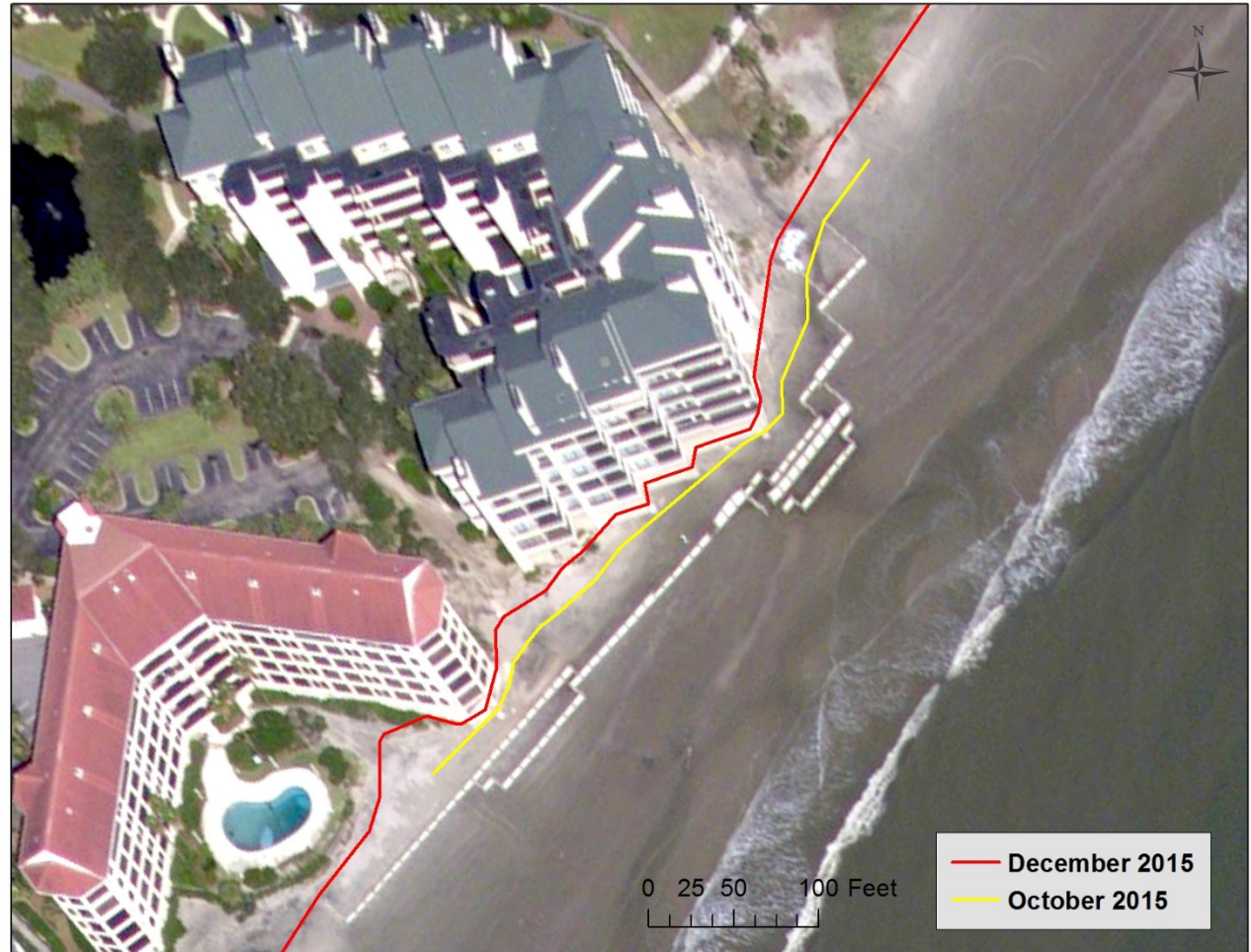
Changes to Scarp Line at Ocean Club and Seascape. OC installation completed June 5, 2015. Seascape installation 1 st tier completed Dec 2015; 2 nd tier completed Feb 2016.
