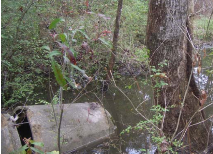
Figure D-3b: Station RS-06027, on Ashby Branch
