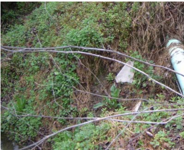
Figure D-3: Station RS-06027, on Ashby Branch
