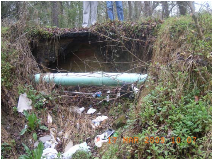
Figure G-3: Station RS-06027, on Ashby Branch. The picture below was taken while standing on the right bank of Ashby Branch depicts area upstream of Clark Street. Note the erosion under the road.
