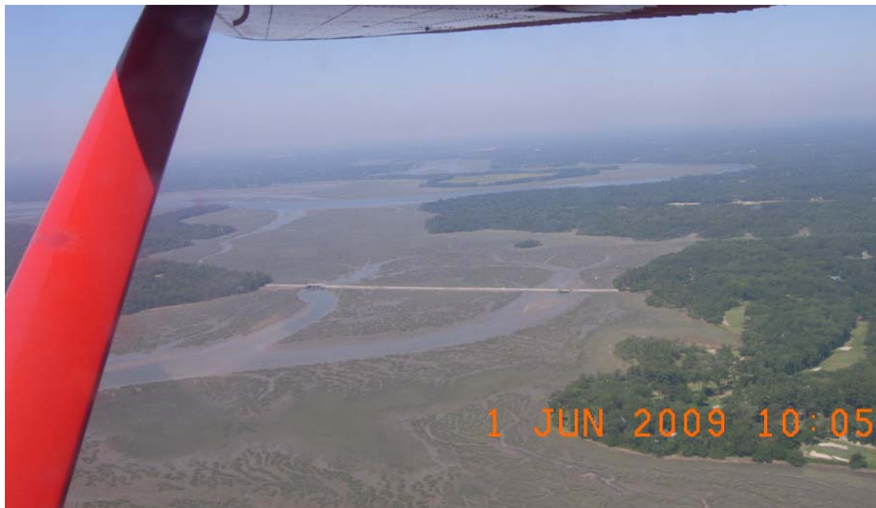
Figure 2. Aerial view of Chechessee Creek and its extensive salt marshes/mud flats. On the right is the mainland and on the left is the Callawassie Island connected with the Callawassie Island Bridge.
