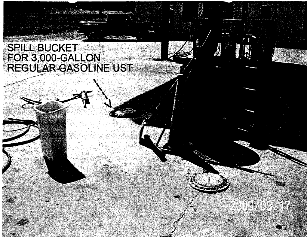
Photograph 1 – View of spill bucket for 3,000-gallon regular gasoline UST.
