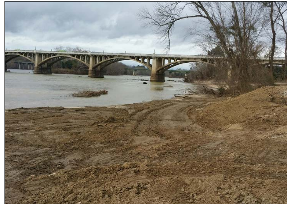
12/14/2015 - Alluvial fan surface restored to post-flood elevations
