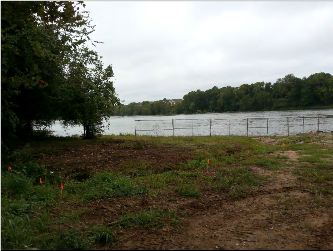
9/2/2015 – View of southern Alluvial Fan from the bottom of the boat ramp.
