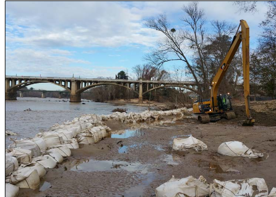
12/07/2015 - Removing sand bags and restoring alluvial fan surface to post-flood conditions
