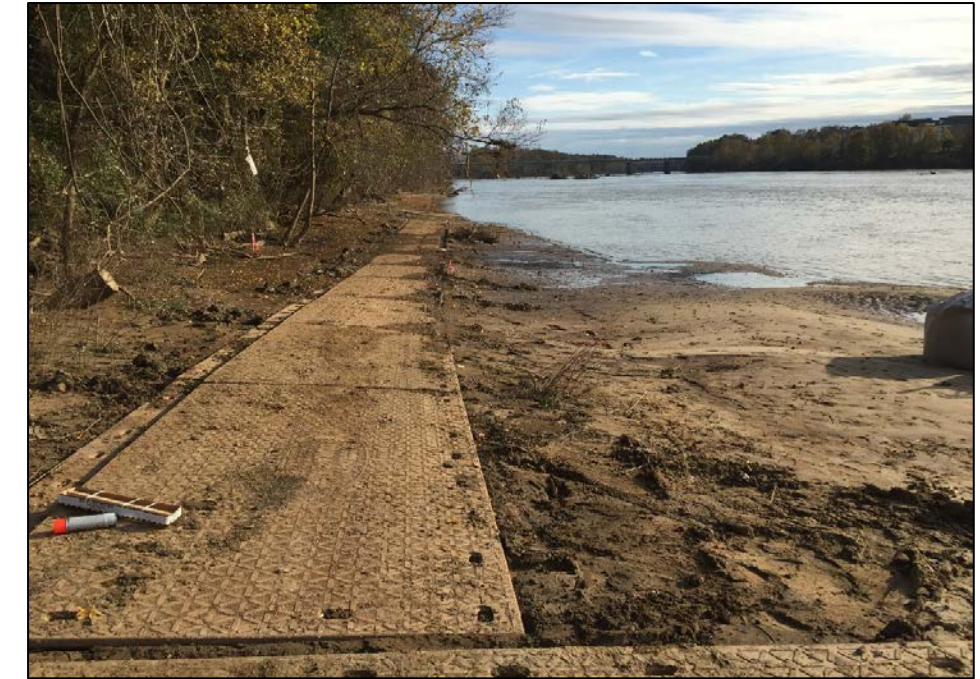
11/17/2015 - Mats deployed along southern alluvial fan to permit access by EOTI
