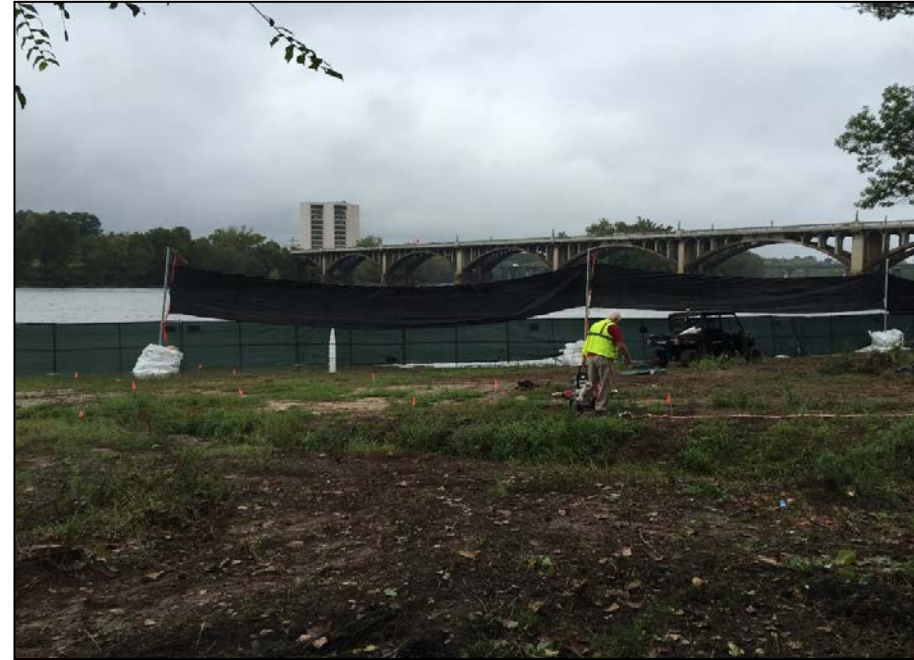
9/29/2015 - Visual barrier installed on northern side of project area
