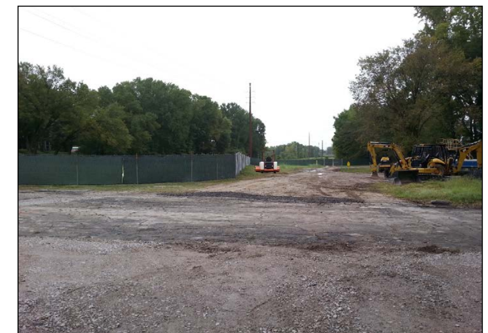
9/28/2015 - Temporary fence with visual barrier & equipment staging
