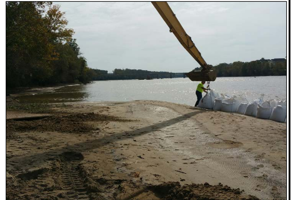
10/29/2015 - Deploying sand bags along river's edge
