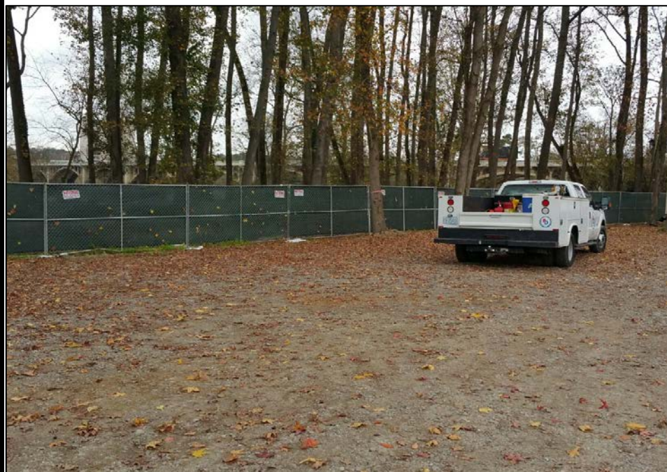
12/14/2015 - Temporary fence placed around trailer compound area
