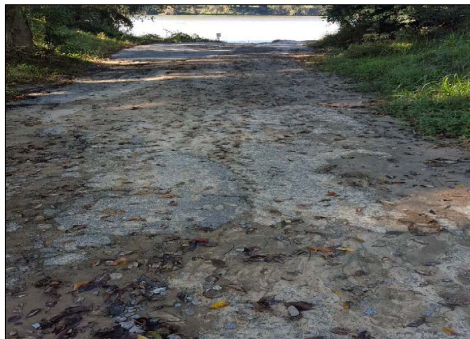
10/19/2015 - View looking down boat ramp
