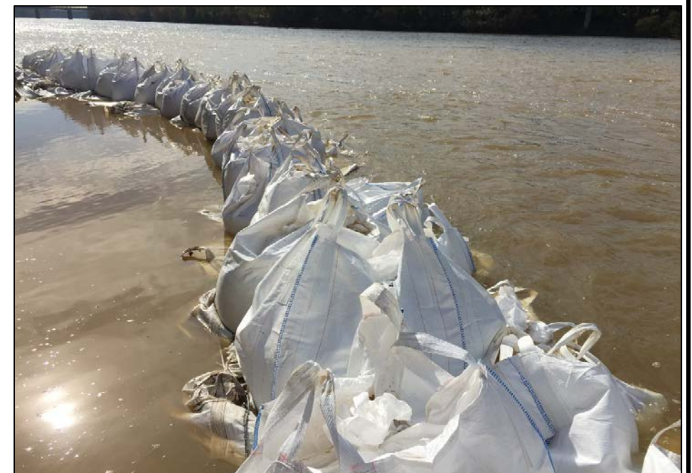
11/17/2015 - Sand bag berm along river's edge
