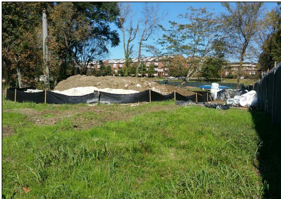
10/30/2015 - Stockpile of sediment removed from alluvial fan area
