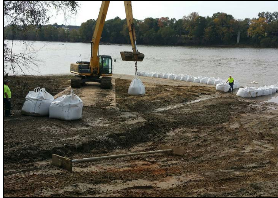
10/29/2015 - Deploying sand bags along river's edge
