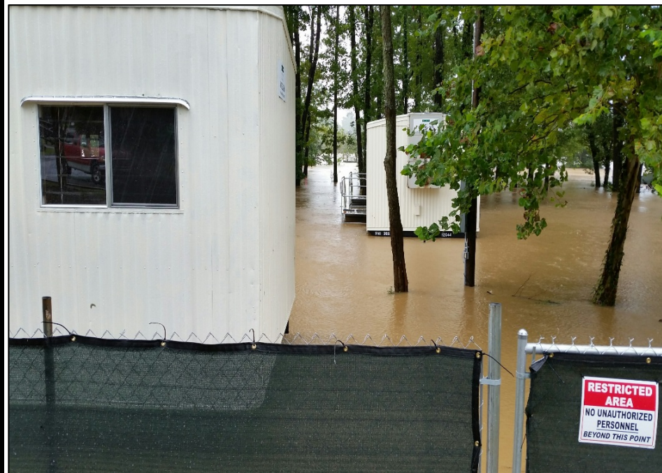
10/04/2015 - Flood waters reaching just below construction trailer floors
