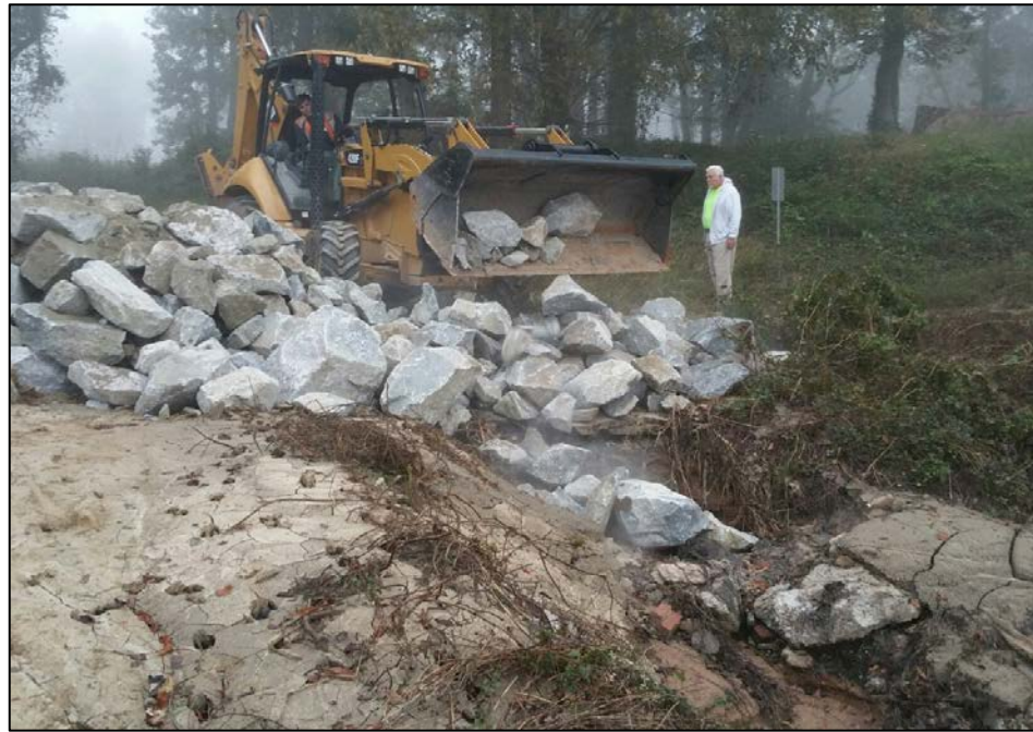
10/23/15 - Stabilizing boat ramp to allow access to alluvial fan
