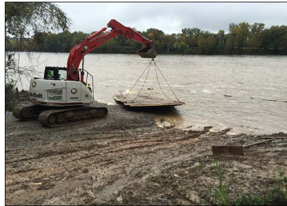
11/2/2015 - Deploying equipment mats to allow access to areas of thick sediment
