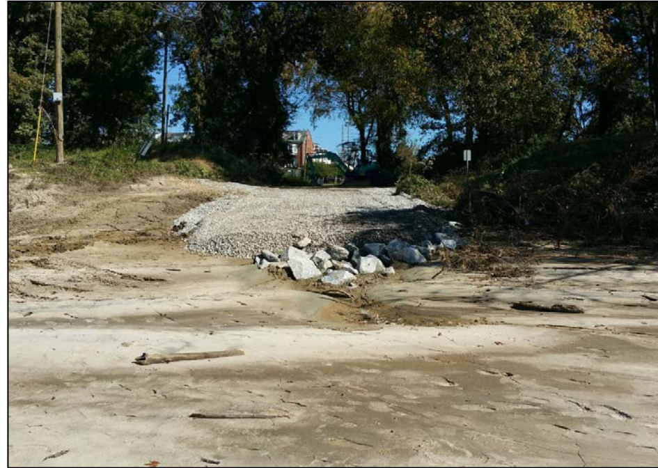
10/23/2015 - Boat ramp stabilized
