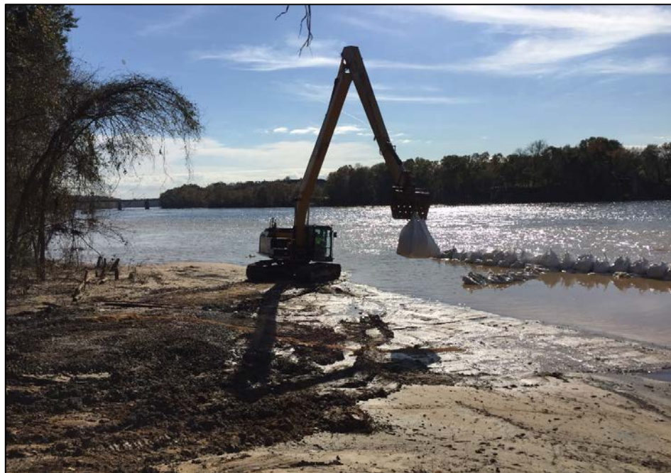
11/16/2015 - Deploying sand bags along river's edge
