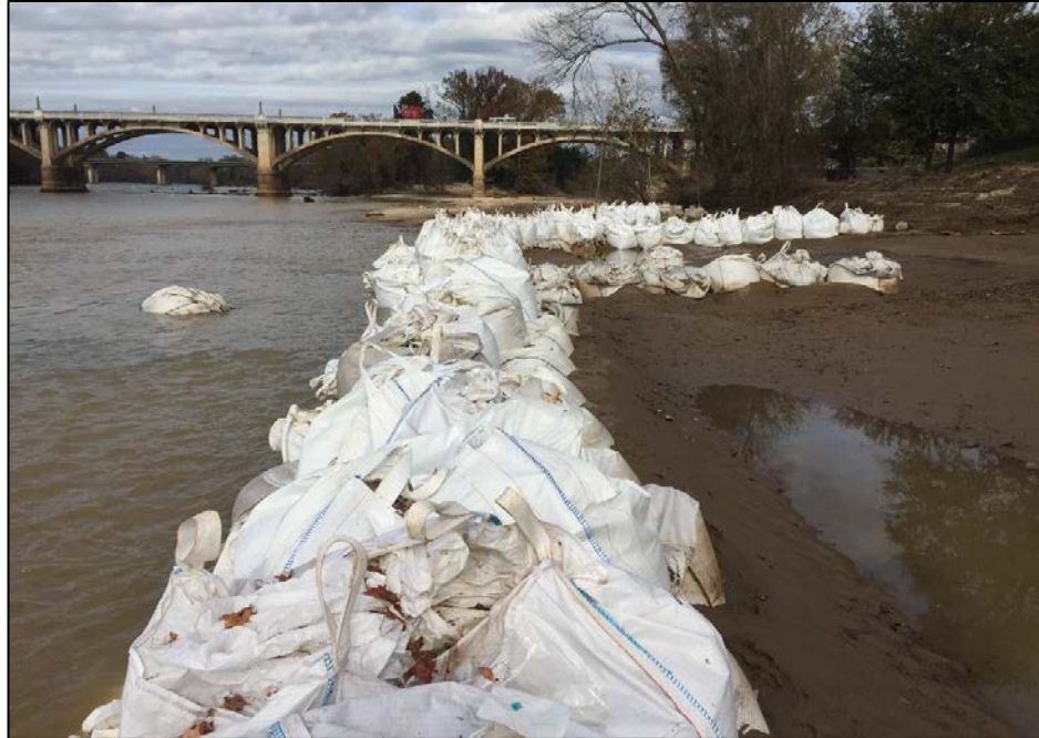
11/17/2015 - Sand bag berm along river's edge
