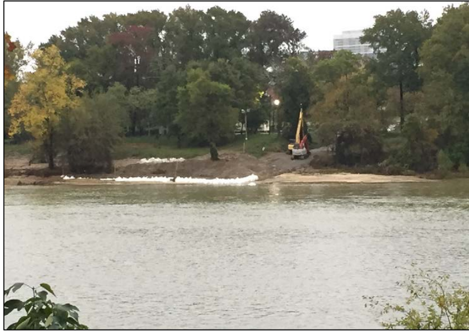
10/27/2015 - View from west river bank of site area with sand bag berm
