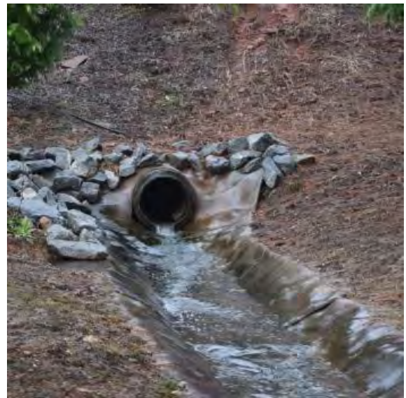
Figure 3: Example of Concrete Cloth in Drainage Channel.
