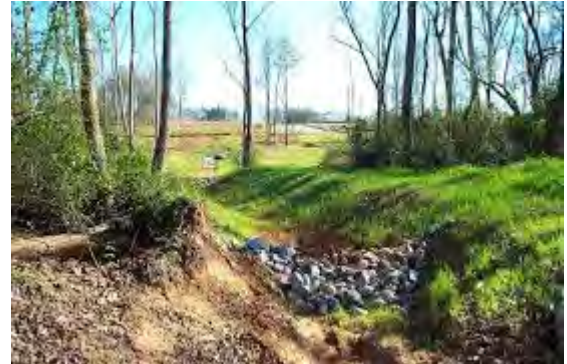
Figure 2: Example Rock Check Dam
