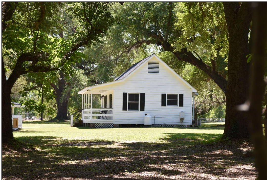
Figure 5.57. Cottage, 75-0314.02, southeast of house, facing southwest.
