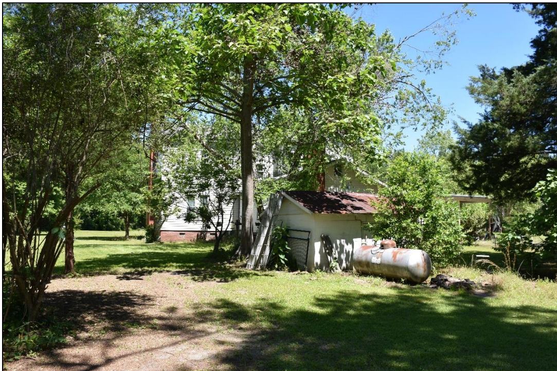
Figure 5.71. Shed (75-0316.03) and rear of house, facing northeast.
