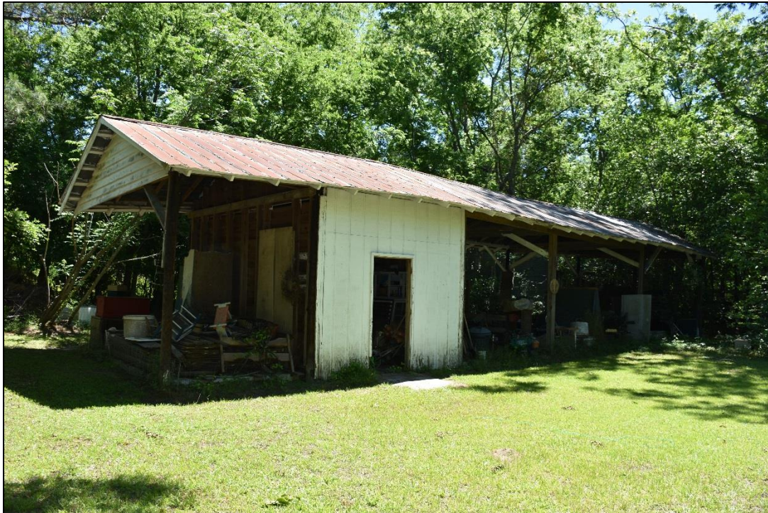
Figure 5.72. Open storage building (75-0316.04), facing southeast.
