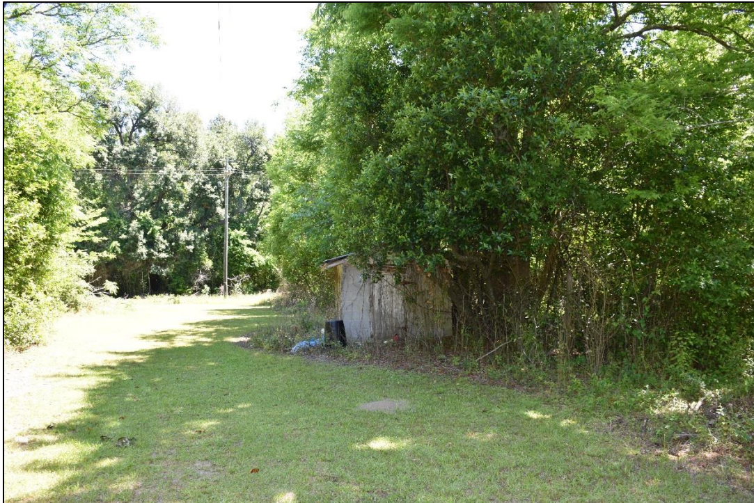
Figure 5.70. Shed (75-0316.02), facing east.
