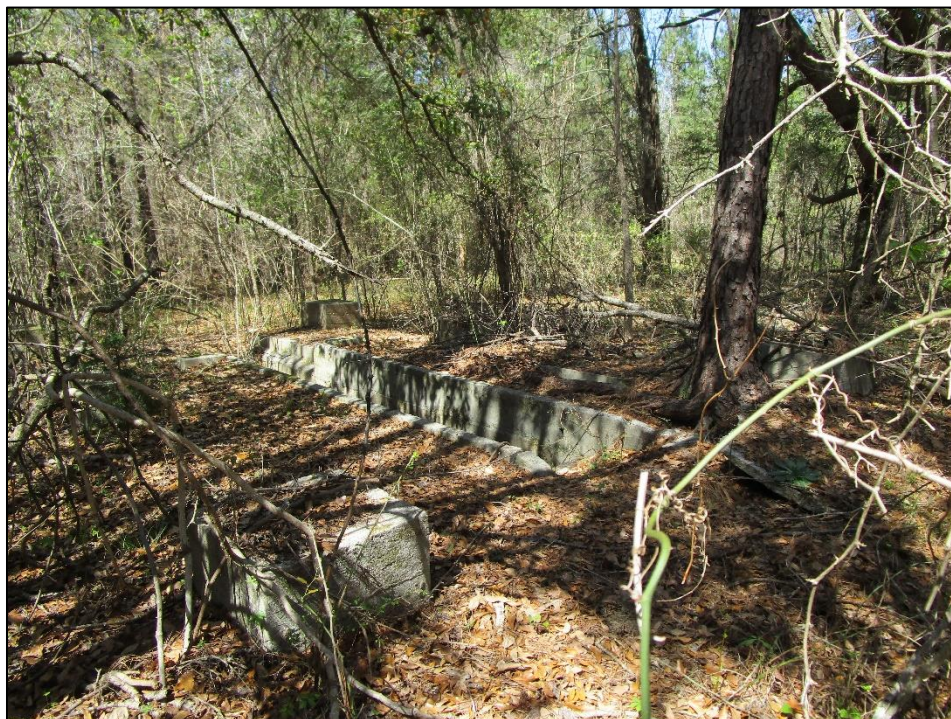
Figure 5.13. Concrete foundation with stairs at site 38OR373 within Area A, facing northwest.
