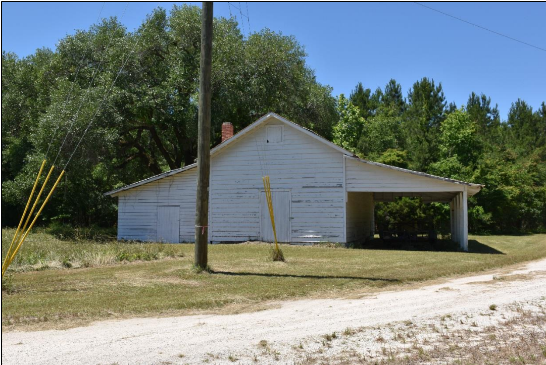
Figure 5.61. Tractor shed (75-0315.01), facing west.
