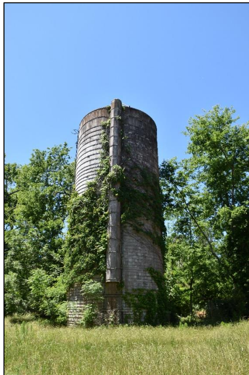
Figure 5.62. Concrete silo (75-0315.02), facing south.
