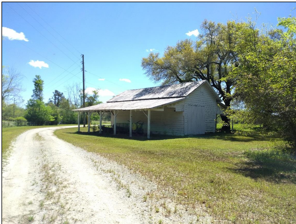
Figure 5.60. Tractor shed (75-0315.01), facing southeast.
