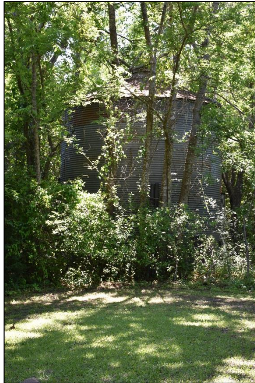
Figure 5.74. Metal silo (75-0316.06), facing south.
