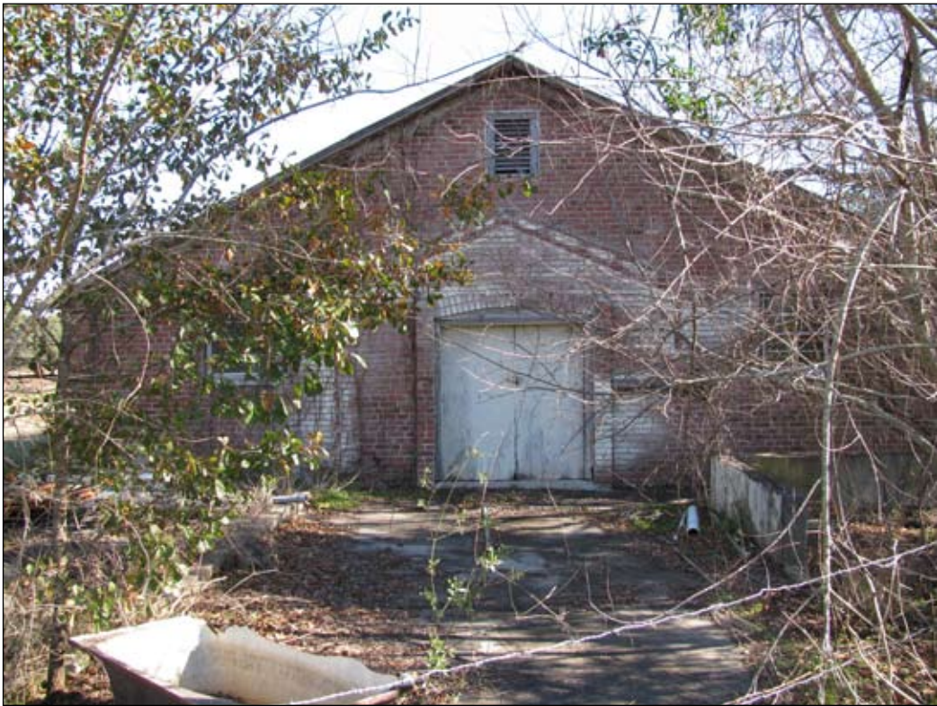
Figure 18. The former milking barn at Walworth.
