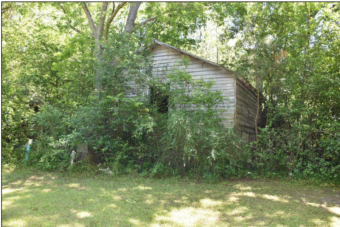
Figure 5.73. Barn (75-0316.05), facing southeast.
