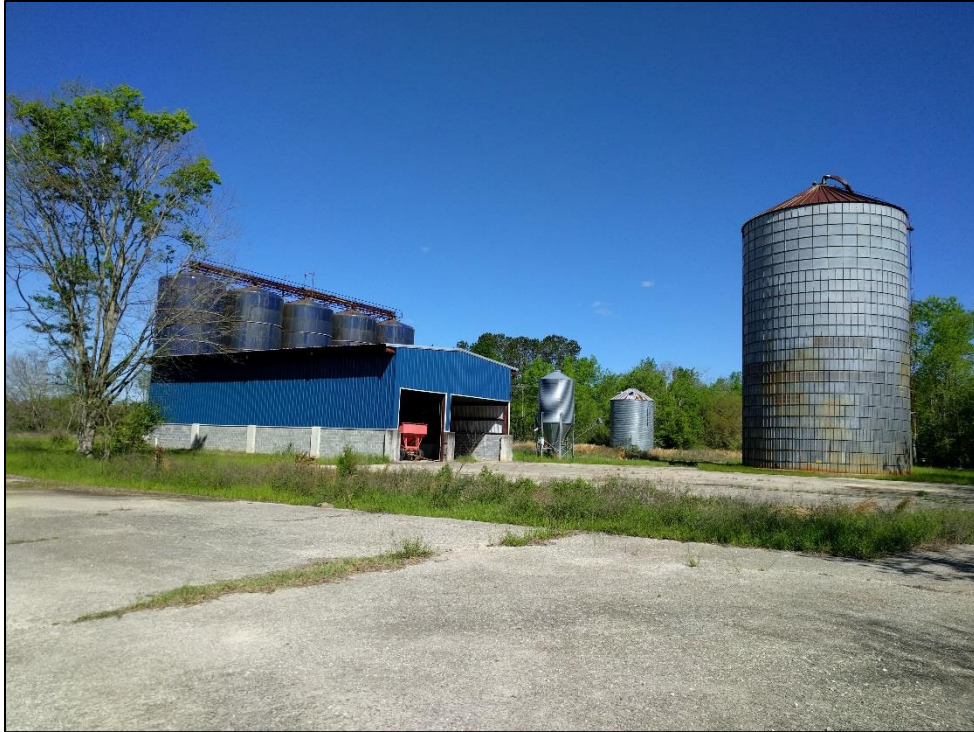
Figure 5.65. Late twentieth century silos and barns, facing east.
