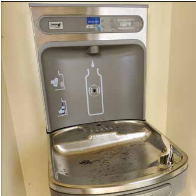
Pictured is a water bottle refilling station. Schools with stations also encourage the use of reusable water bottles.
