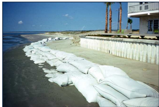
FIGURE T-4. Shore-protection structures at the Beach Club in September 1974 prior to the club's opening.
